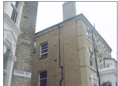
Gutters and downpipe
