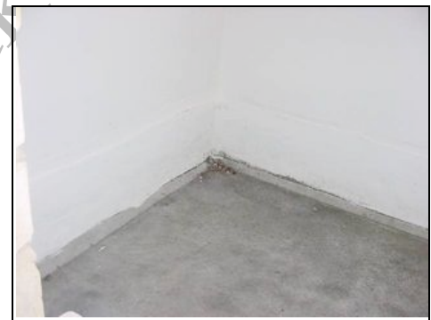
Flat roof entrance area
