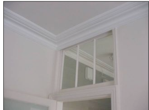
Ornamental plaster ceiling and coving
