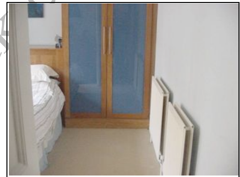
Radiators not next to a window
