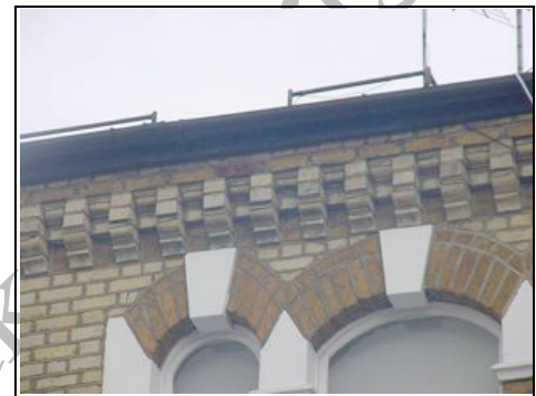
Close up of brick corbelling
