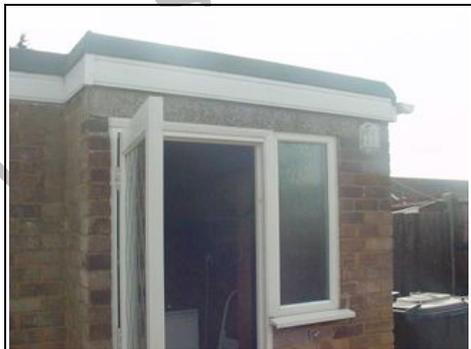
Example of a concrete lintel – can you notice where the cold bridging would be in this photo?
