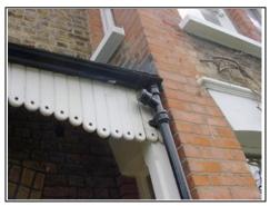
Unusual cast iron downpipe on the front roof with extra branch on the downpipe
