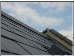
Slipped tile to left hand parapet wall
