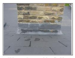
Chimney One requiring flashing to be correctly bedded into brickwork
