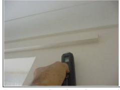
Dampness and condensation around the concrete window lintel
