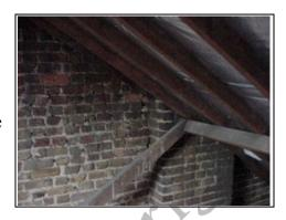
General view of inside of roof showing common rafters (ones that form the pitch of the roof) purlins, cross brace and brace to the central wall.
