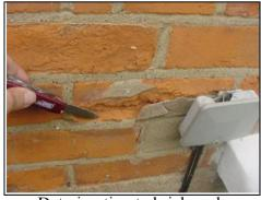
Deterioration to brickwork incorrectly re-pointed in cement mortar rather than lime based mortar 42
