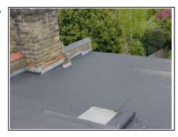
Roof light partly felted over
