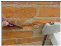
Deterioration to brickwork incorrectly re-pointed in cement mortar
