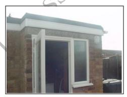
Example of a concrete lintel – can you notice where the cold bridging would be in this photo?
