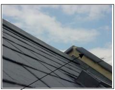
Slipped coping stone to left hand side parapet wall
