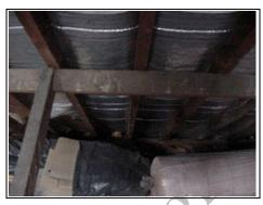
This photo shows the common rafters (the ones that form the pitch of the roof) and the silver area between is the protective underlayer.
