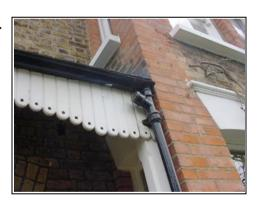
Unusual cast iron gutter and downpipe to the front roof with extra branch
