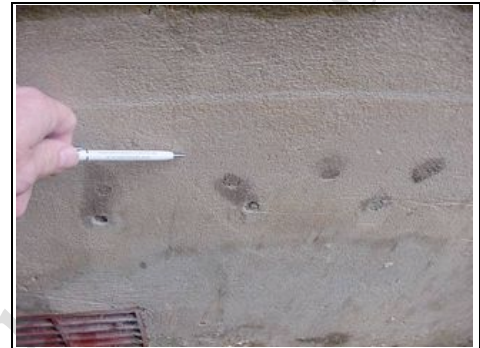
Damp proof course has been inserted on the left hand side
