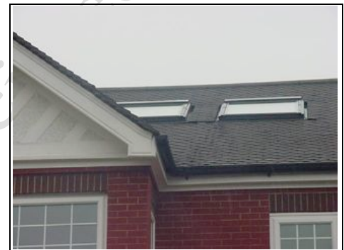
Fascias and soffits
