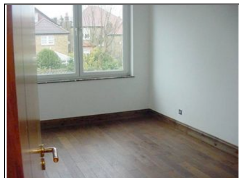
Rear room on right hand side
