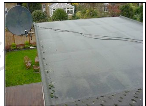
Flat roof to rear of property
