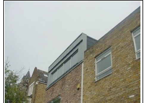
Stretcher bond brickwork
