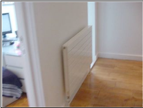
Internal radiators should be moved underneath windows
