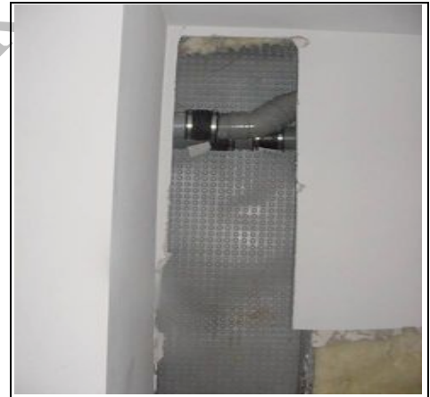
Leaking joint
