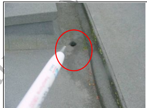
Small outlet on main roof
