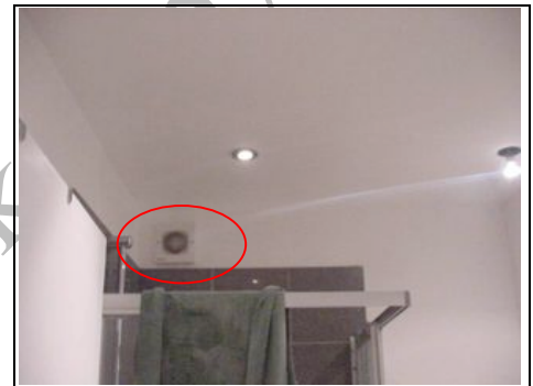
Replace with large humidity controlled extract fans
