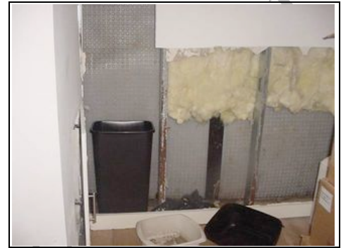
We can see the tanking/damp proof membrane in place.
