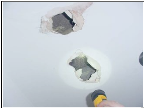
Opening up ceiling to resolve problems with traps
