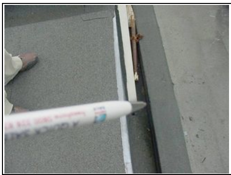
Box gutter on flat roof
