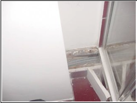
Plastic pipes in lower ground floor
