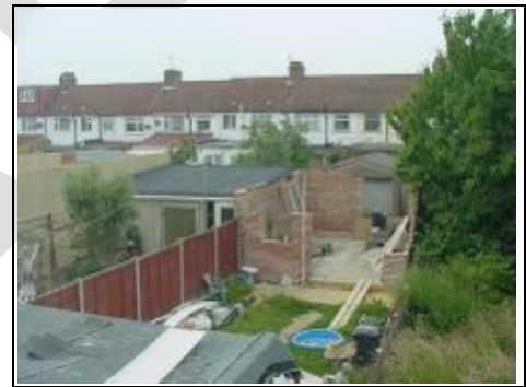
Left hand neighbour's garage/storeroom
