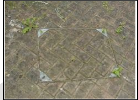
Manhole two (rear)
