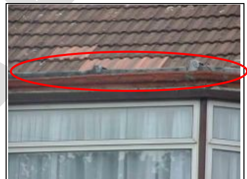
Flat roof to bay window
