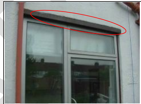
Timber sill forms the drip detail
