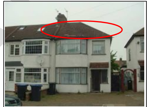
Main hipped roof
