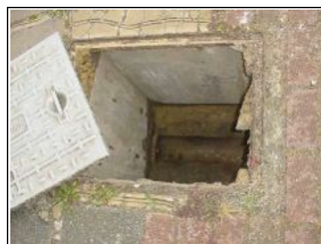
Manhole one (front right)
