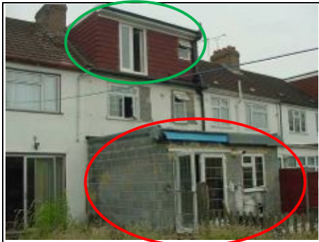
Neighbours rear extensions are on the party wall
