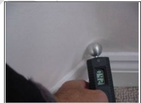
Testing for rising damp
