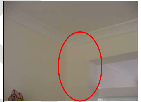
Wall removed with pier support
