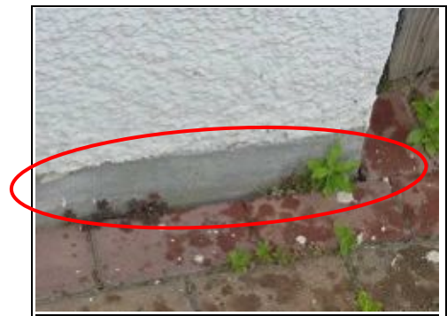
No bell mouth but this detail to the base of the render can draw water into the property
