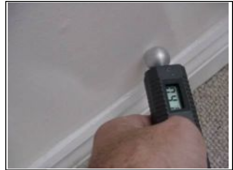
Checking for dampness
