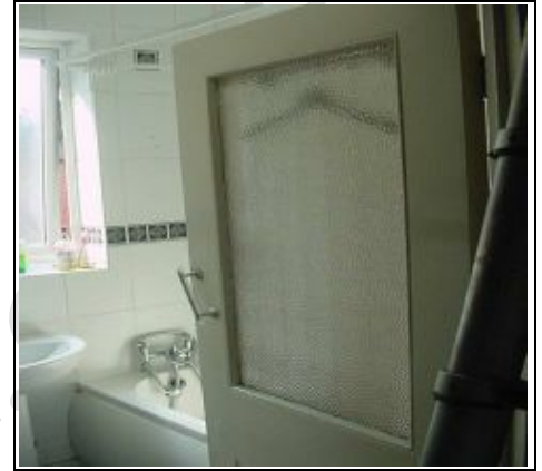
Glazed door to bathroom
