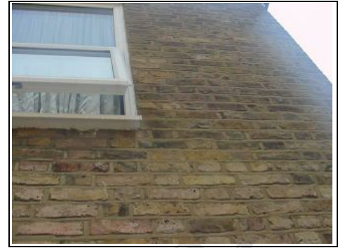
Bricks re-pointed in cement mortar
