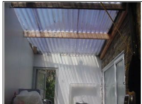
Plastic lean-to roof
