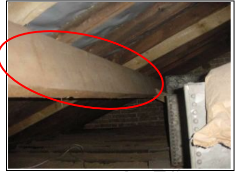
New purlin added
