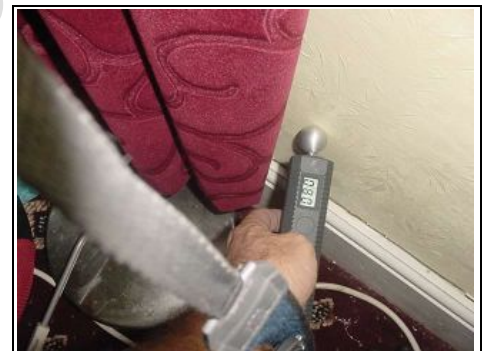
Testing for rising damp
