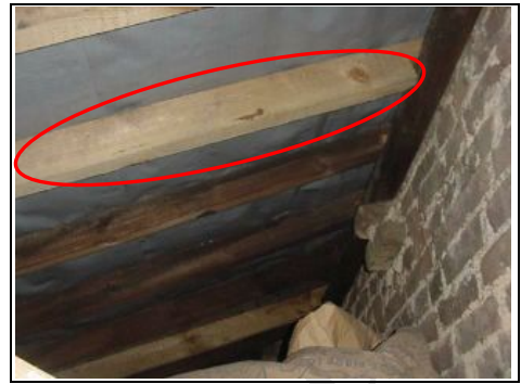
New timbers added in rear roof
