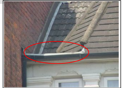
Flat roof (front left)
