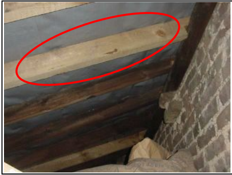
New common rafters have been added
