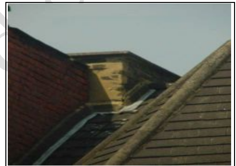
Chimney (front left)
