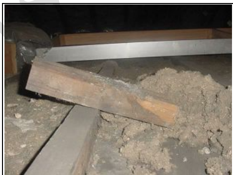
Main roof has older style insulation
