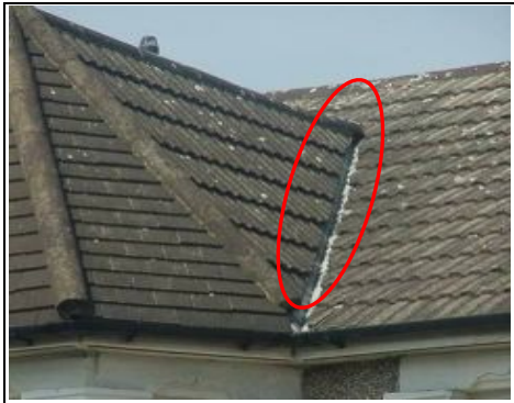
Thin valley gutter
