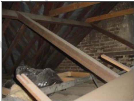
Cut timber roof with timbers added
