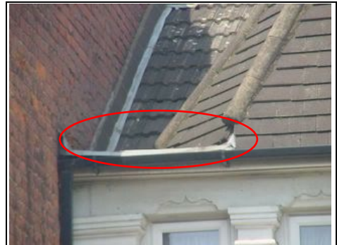
Flat roof section
