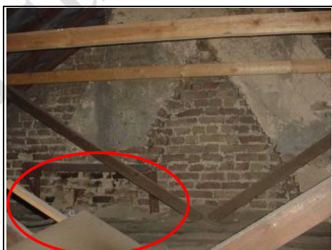
Chimney removed and supported by gallows brackets
