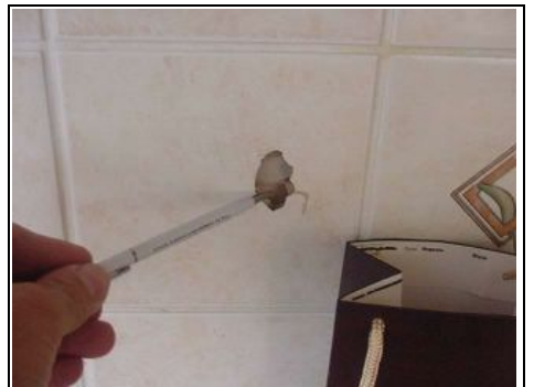
The walls in the kitchen have been dry lined
