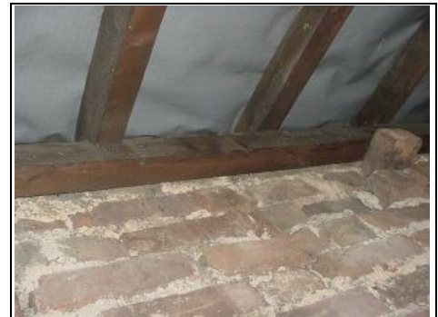
Older timbers show minimal cuts
