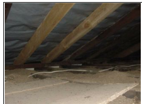
Fibreglass insulation in the rear roof
