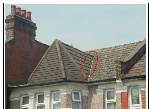
Narrow valley gutters
