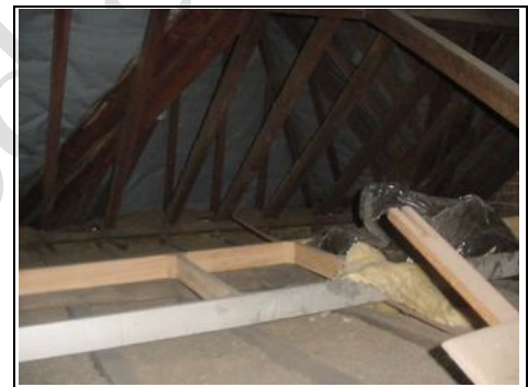
General view of inside of main roof
