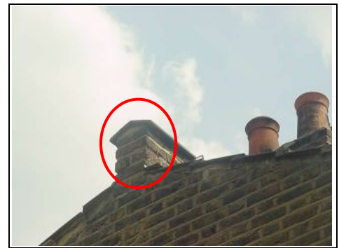
Rear parapet wall
