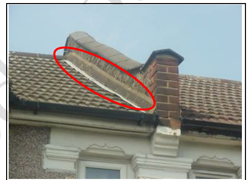
Front right parapet wall with tile on edge flashing
