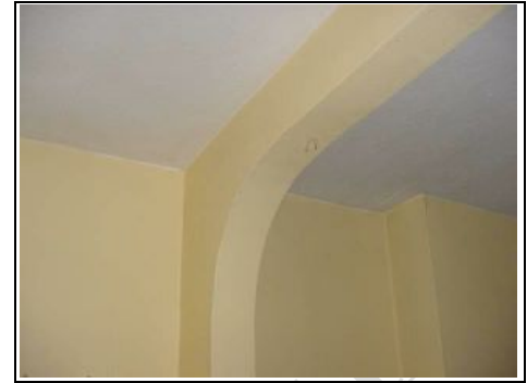
Wall removed in lounge
