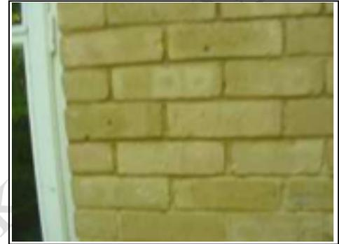
Stretcher Bond brickwork
