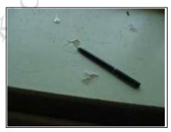
Peeling paint noted on the window sill- this is a sign of condensation
