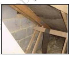
This photo shows the common rafters (the ones that form the pitch of the roof) and the dark area between is the underlayer
