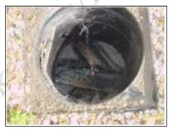
Water was slow to run away from the drains, in fact water sat in the drains
