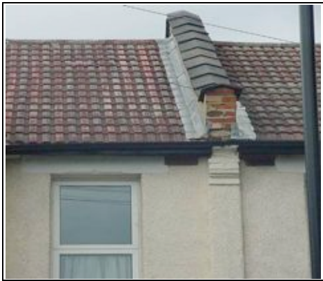
Parapet wall (left)
