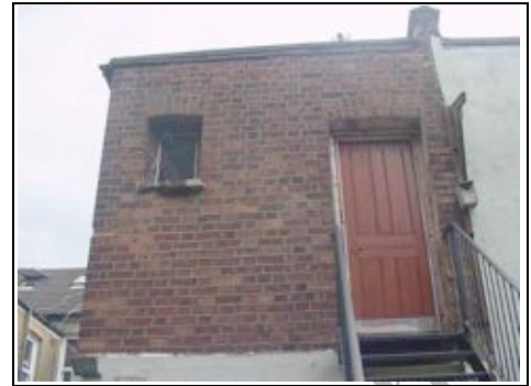
Brickwork at first floor level
