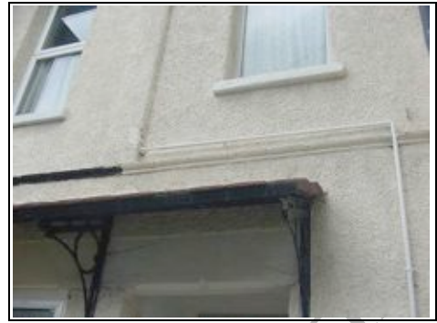
Small canopy over the front door
