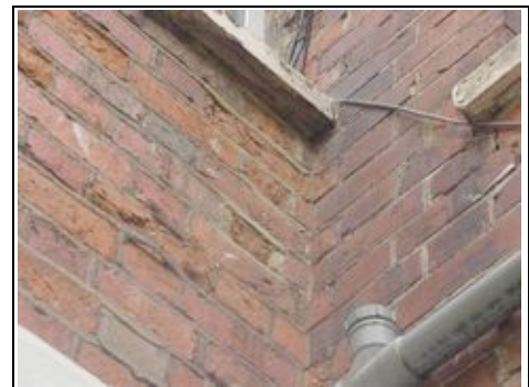
Spalling brickwork
