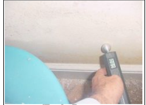
Testing for dampness
