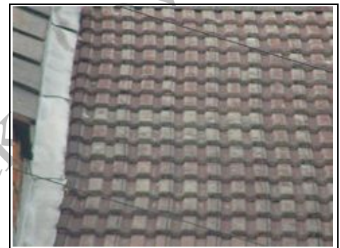
Concrete tiles on main roof
