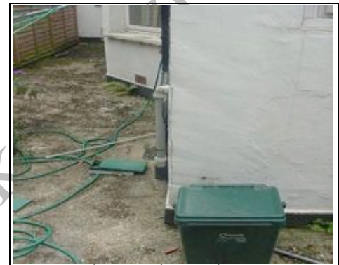
Render repairs to the rear right corner
