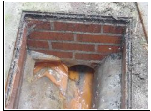
Manhole two (rear)
