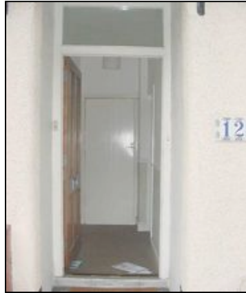
Entrance door and lobby
