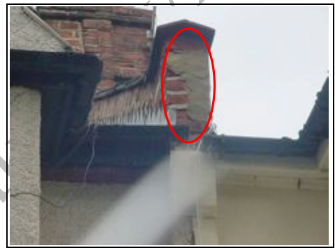
Parapet wall (right)
