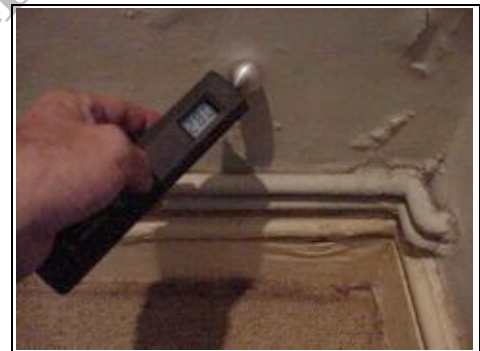
Testing for rising damp
