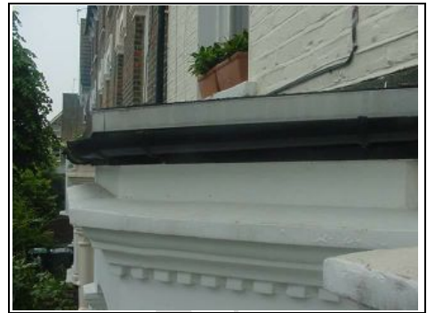
Bay window roof
