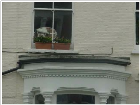
Flat roof over the bay window
