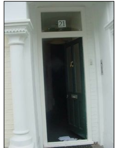
Front entrance door
