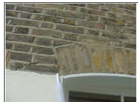
Bricks re-pointed in cement mortar
