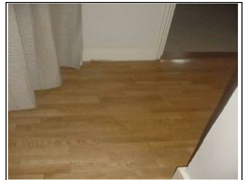
Laminate flooring hiding the floor beneath
