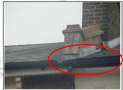
Gutter and downpipe
