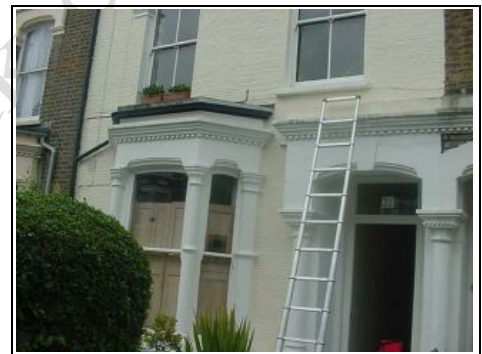
Inspecting the roof
