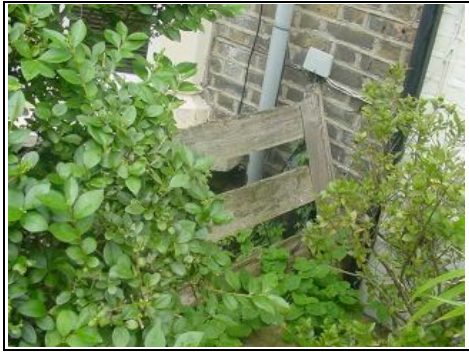
Fence missing front left hand side
