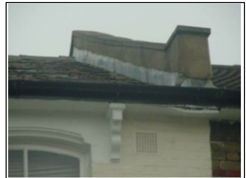
Parapet wall (front right)
