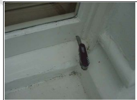
Knife test to window
