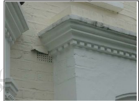
Painted Flemish Bond brickwork
