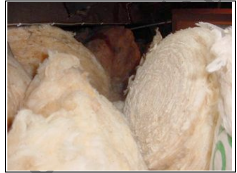
Bundles of excess insulation
