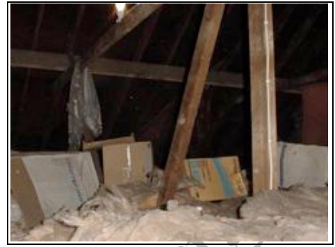
General view of inside of roof
