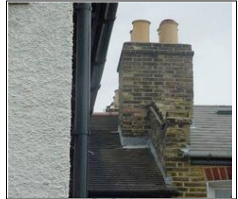
Rear left chimney
