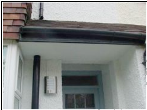
Porch roof over front entrance
