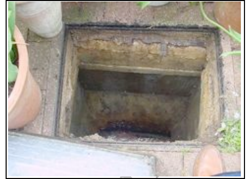
Manhole two- rear
