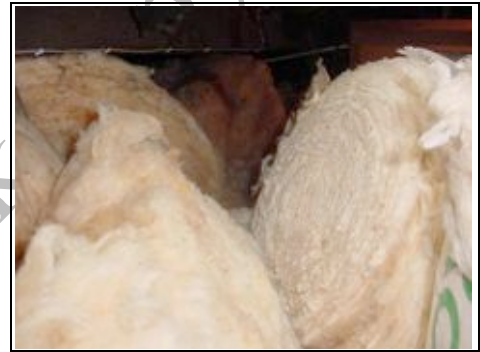
Bundles of insulation. This is the problem when you pay for an amount of insulation rather than for it to be installed properly
