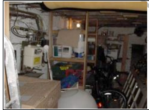
General view of cellar
