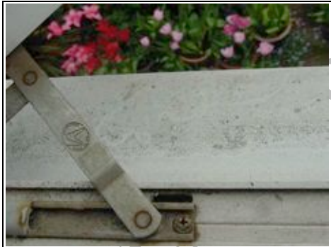
Ingrained dirt to plastic windows
