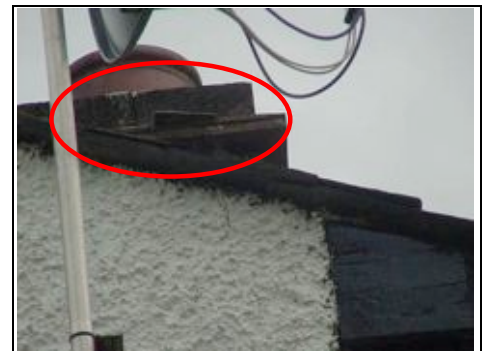
Only the chimney pot is visible
