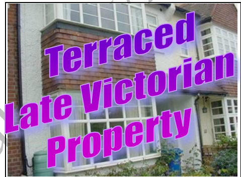
Painted roughcast render and vertical tiling
