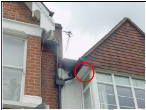
Fascias and soffits
