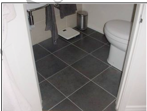
Tiles laid on a timber floor
