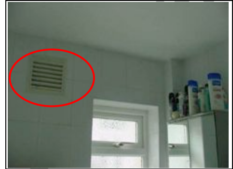
Air vent at high level
