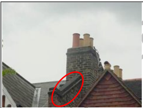
Front left parapet wall
