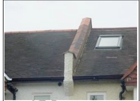
Front right parapet wall
