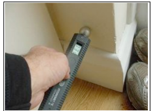
Testing for rising damp
