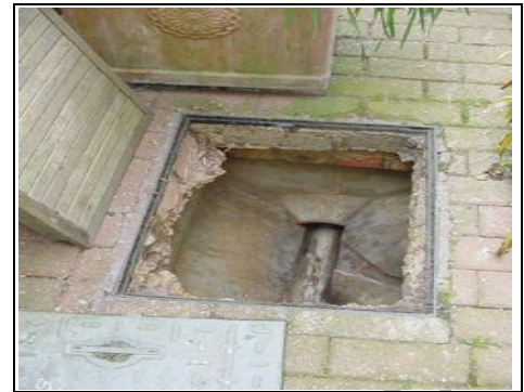
Drain is concrete, which can indicate work has taken place to the drains
