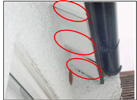
Exposed rafter feet
