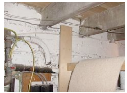
Timbers embedded in the walls
