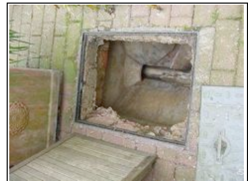
Manhole one- rear left
