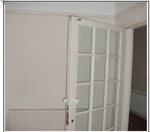
Glass door without kite marks to glass
