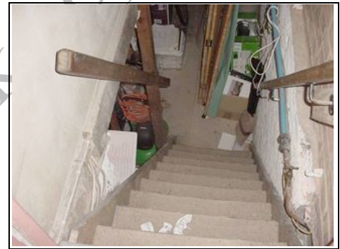
Looking down into the cellar
