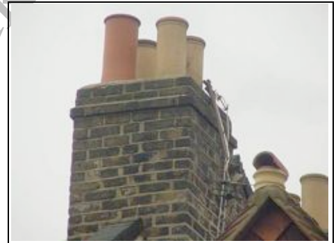
Chimney- front left
