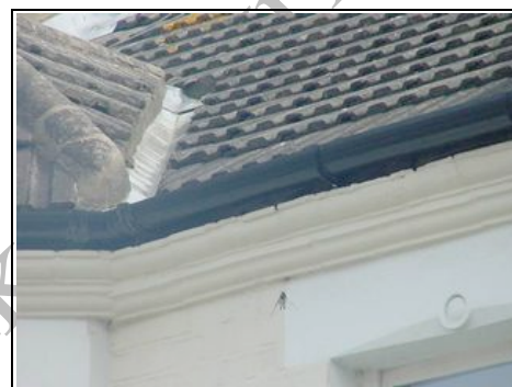
Sit over guttering with tile on edge
