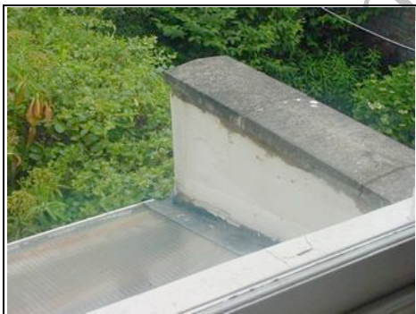
Rear parapet wall
