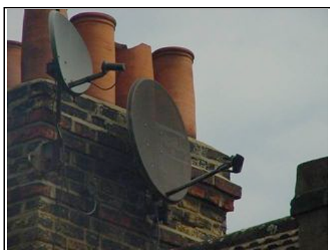
Chimney to front left
