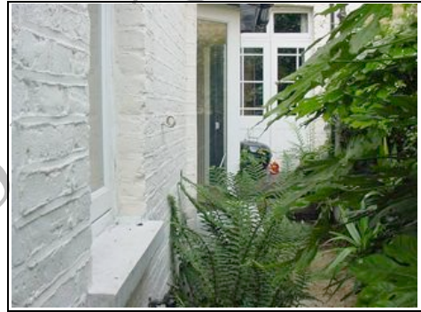
Rear view looking down
