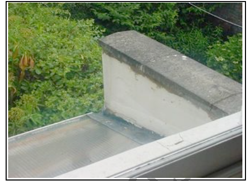
Polycarbonate roof to rear
