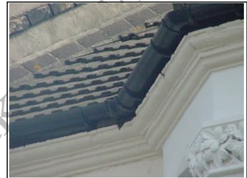
Fascias and soffits
