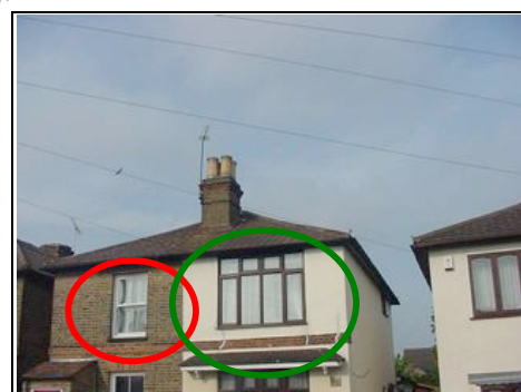
Victorian property that has been modernised Red oval is original sliding sash window Green oval is new large window that has been added
