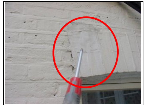
Repairs to soldier course above window
