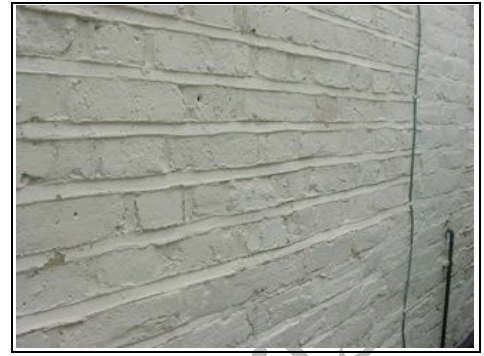
Cement mortar pointing
