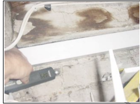
Checking for dampness in the cellar
