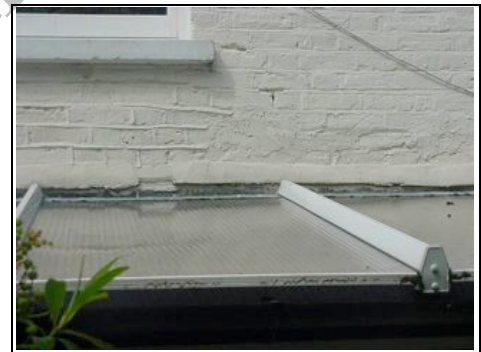
Polycarbonate roof to rear
