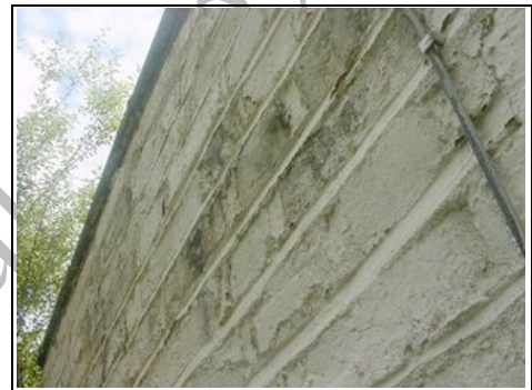
Coping stone is not large enough and there is no drip detail
