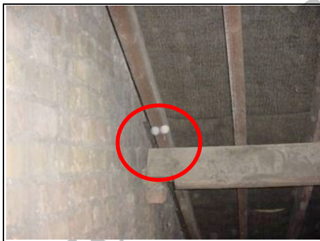
Purlin – delicately positioned on bricks
