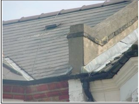
Parapet wall to front left side
