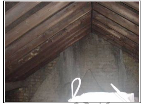
General view of inside of roof
