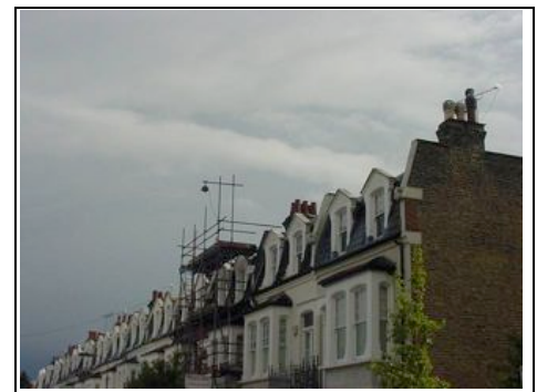
Loft conversion and dormer windows
