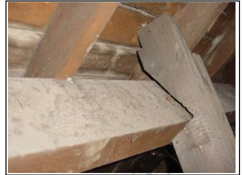
Timbers to props cut too deeply known as a bird mouth
