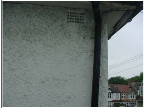
Roughcast render with patches of repair
