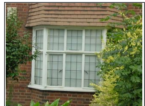
Metal Crittall can suffer from cold bridging
