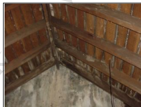
Dampness around chimney
