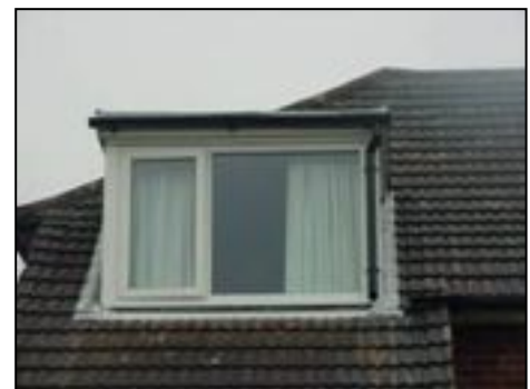
Heat can be lost through a dormer window in the roof
