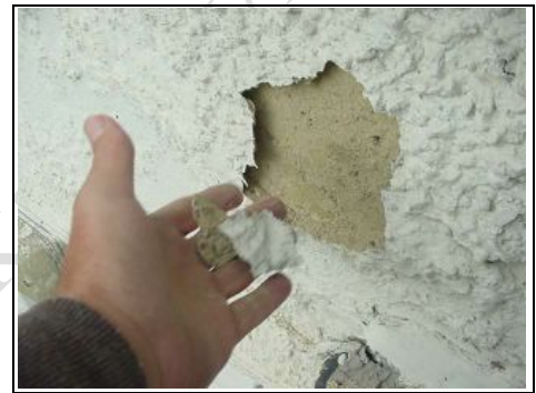
Deterioration to render
