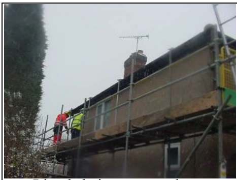
Lintels being removed on 1930's/1950's house
