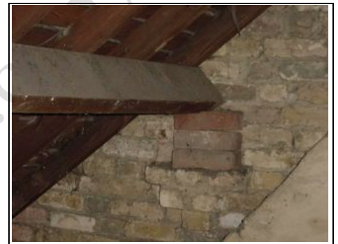
Purlins balanced on bricks to the rear
