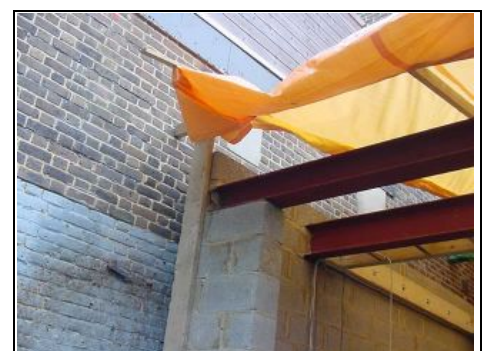
Outside detailing of metalwork onto blockwork
