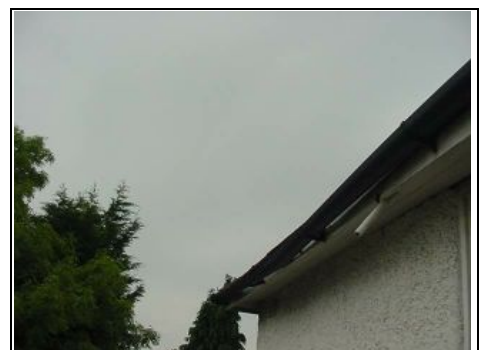
Twist/drop in the gutter
