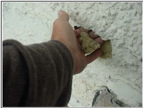
Deteriorating render
