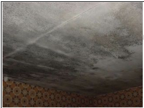
Ceiling covered in black mould
