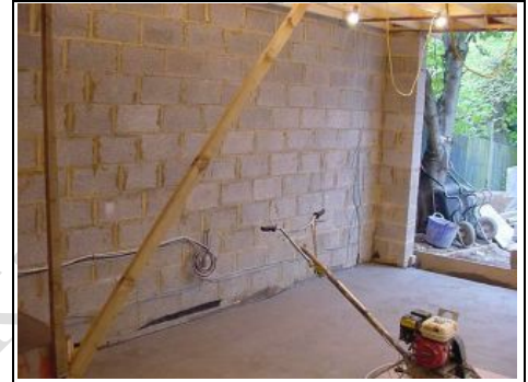
Looking towards the party wall, we are advised the builder has used a sound block
