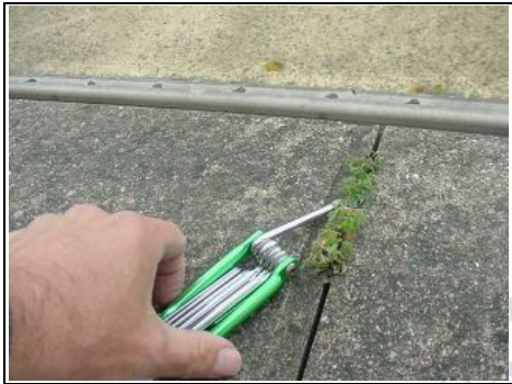
Parapet wall is letting water in
