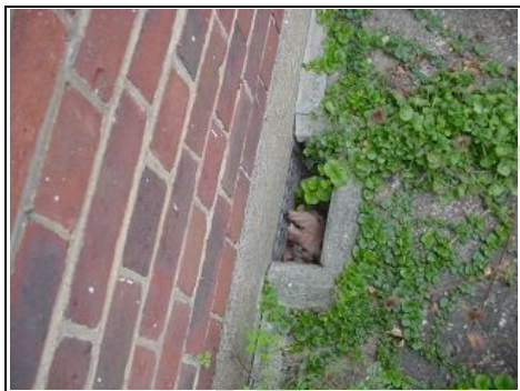
Air vent to front. High ground level
