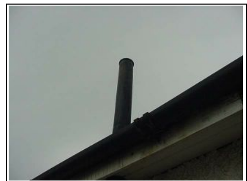
Soil and vent pipe
