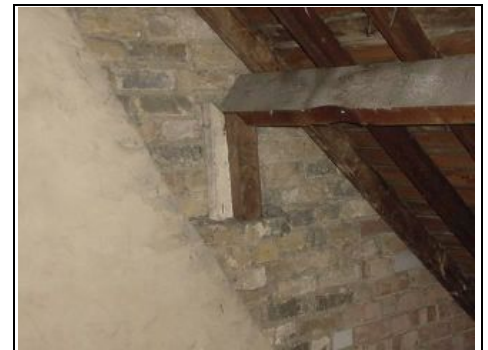
Purlins balanced on timber to the front
