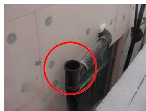
Old soil and vent pipe replaced with plastic
