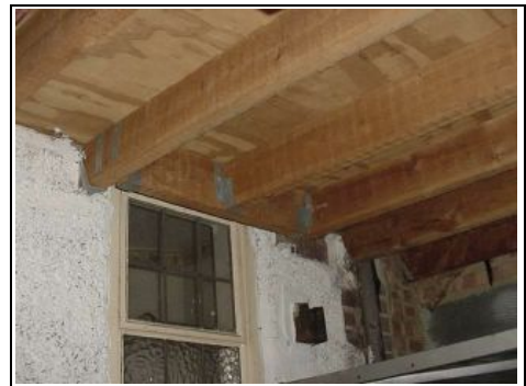
Joist hangers to underside of garage roof indicating it is relatively new
