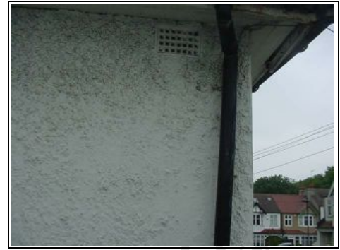
Roughcast render repaired with areas of smoother render.
