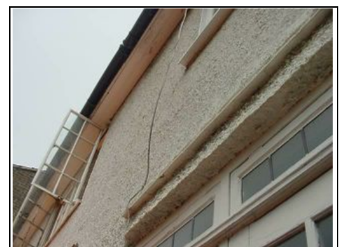
Drip details in render formed by tiles
