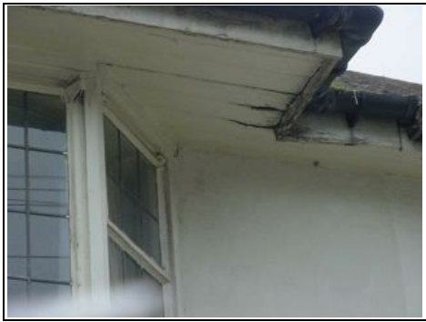
Fascias and soffits deteriorating due to leaking gutters!
