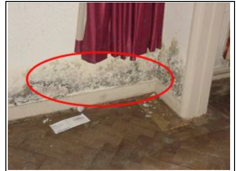
Mould caused by cold bridging
