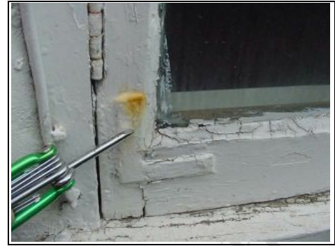
L brackets on windows indicating they have deteriorated
