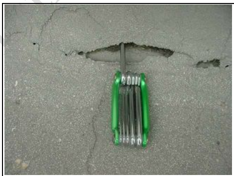
Holes to asphalt roof
