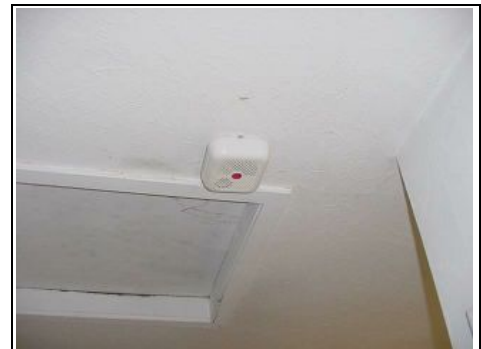
Battery operated smoke alarm needs improving
