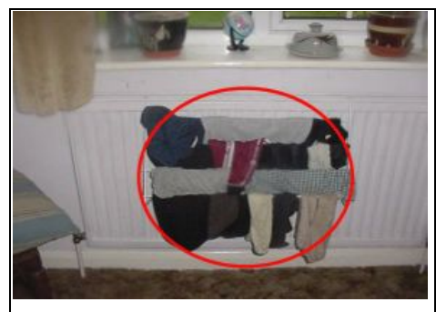
Washing drying on radiators creates moisture
