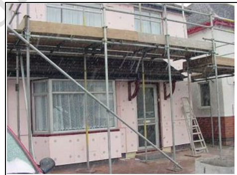
External wall insulation
