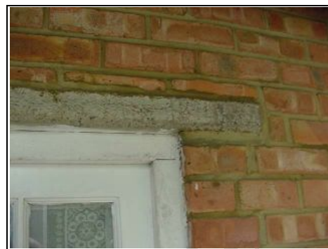
Concrete lintels
