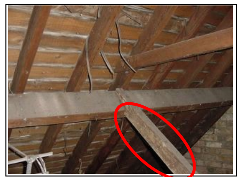
Thin strut supporting purlin
