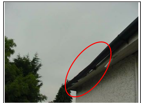
Guttering dropping to left side
