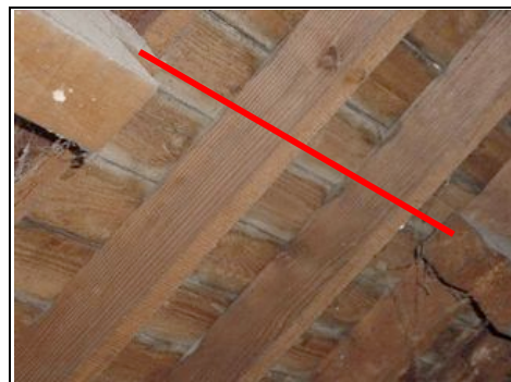
Cut purlin – the red line shows where the purlin should be
