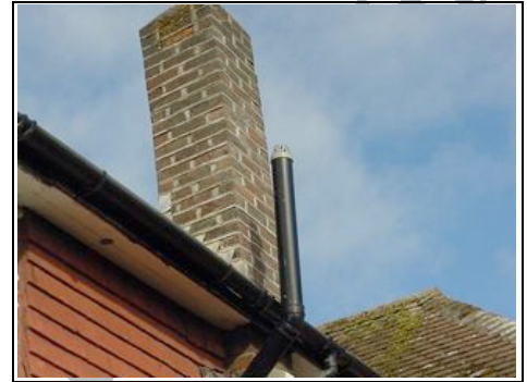
Rear plastic soil and vent pipe
