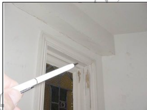
Water damage in shower room in annexe which may be partly condensation and partly a roof leak
