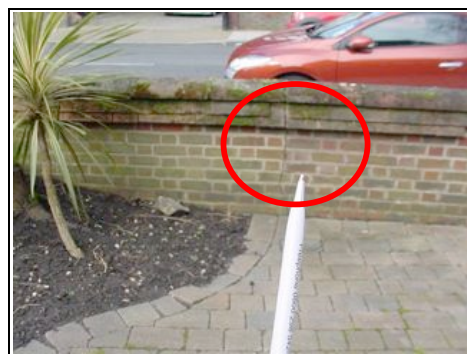
Crack to front brick wall where tree has been removed
