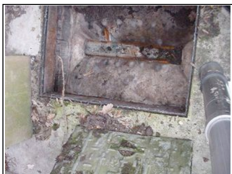
Front right hand manhole appears to be blocked
