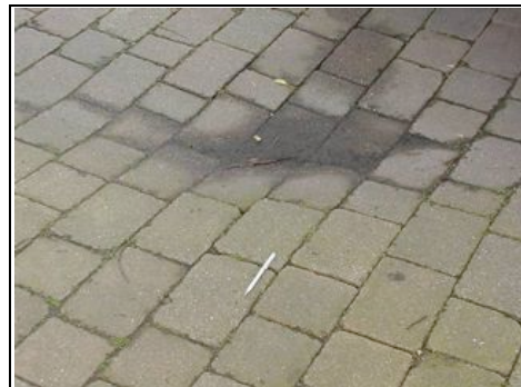
Dip in pavia slabs
