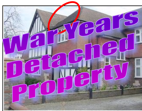
Valley gutter – where one pitch of the roof meets the other
