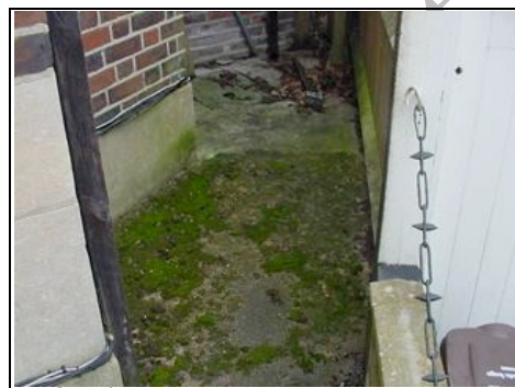
Area of moss on the right hand side indicates there is possibly a leak from the supply pipe/drainage and there is a manhole cover nearby
