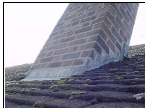
Close up of lead flashing and brickwork of front left hand chimney
