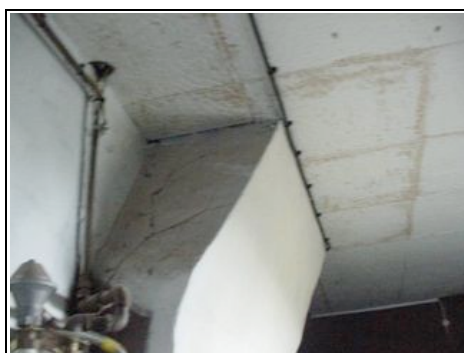
Polystyrene tile to ceiling in garage which needs removing
