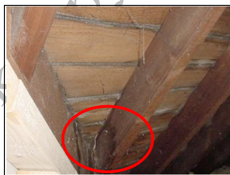
View front left hand roof with dampness coming through
