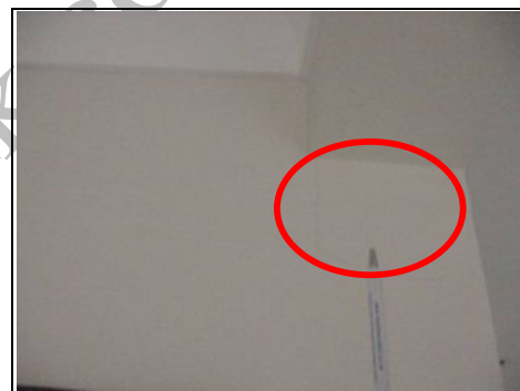
Resulting hairline cracking in hallway
