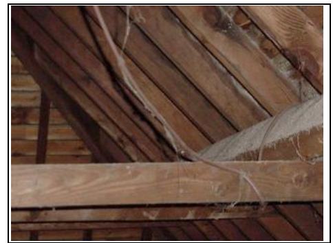
Dampness coming into the roof on the timbers
