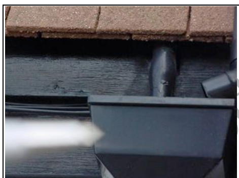
Possible lead pipework externally
