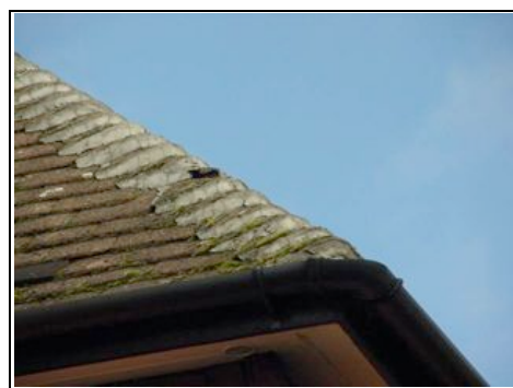
Hipped ridge has been re-bedded
