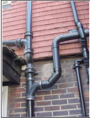
Left hand side cast iron and plastic soil and vent pipe
