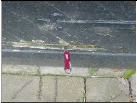
Knife test to garage door
