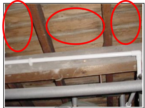
Dampness coming in to front left hand roof
