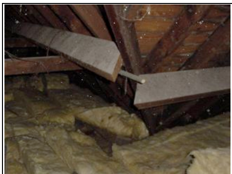
We would have expected support, particularly to the right hand purlin
