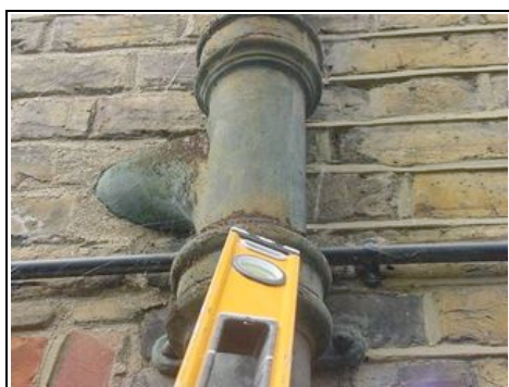
Rusting soil and vent pipe
