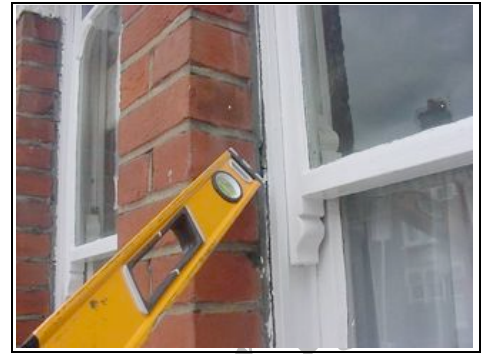
Cracking around window
