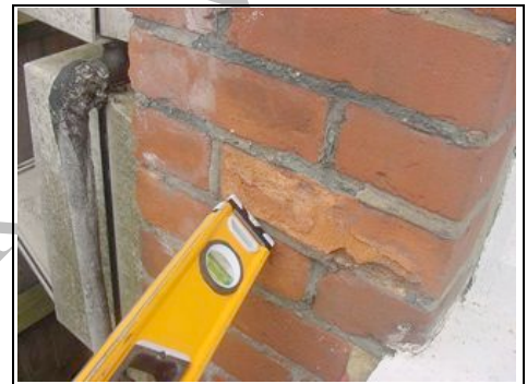
Spalling to brickwork
