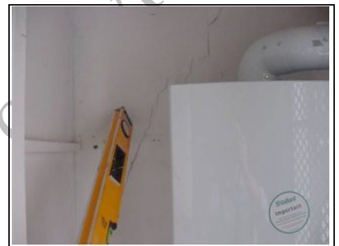
Crack in boiler cupboard
