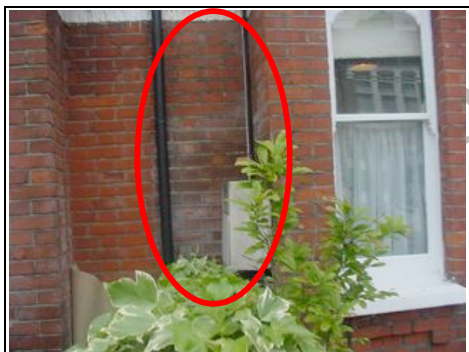
Dampness to brickwork
