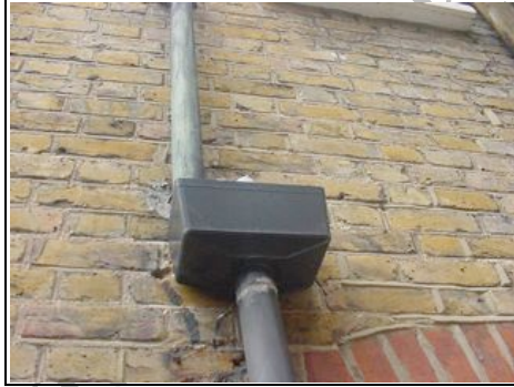
Overflowing hopperhead
