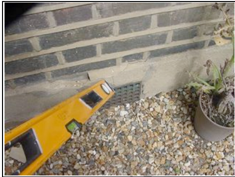
Airbrick acting as gutter
