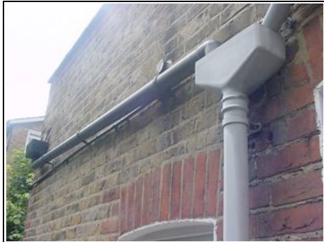
Gutters and downpipes
