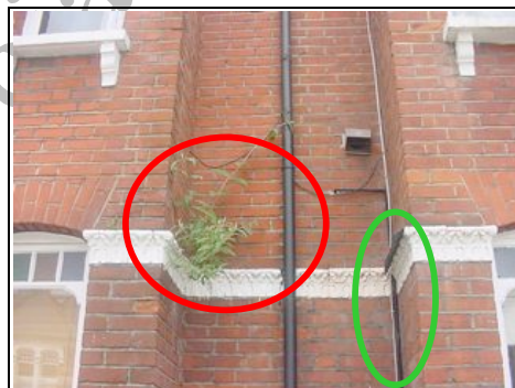
Plant growing the top of the coade stone (red), felt detailing added (green)
