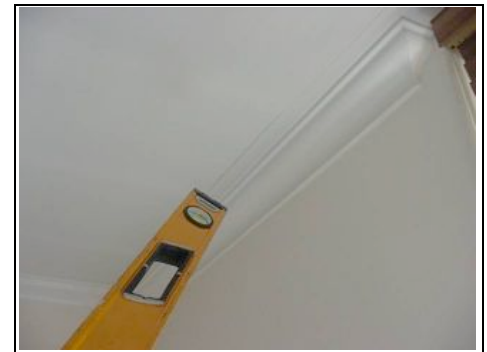
Hairline cracks to rear part of property, which could be due to dampness
