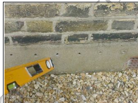
Inserted damp proof course to rear unnecessary
