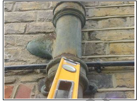
Rusting soil and vent pipe
