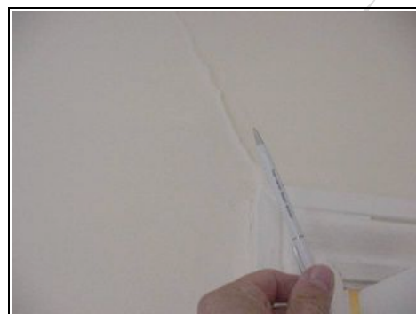
Movement visible to front bedroom above door
