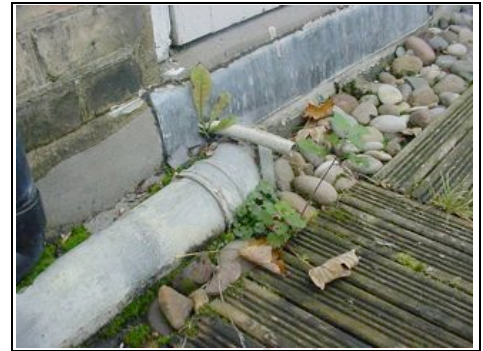
Soil and vent pipe awkward run
