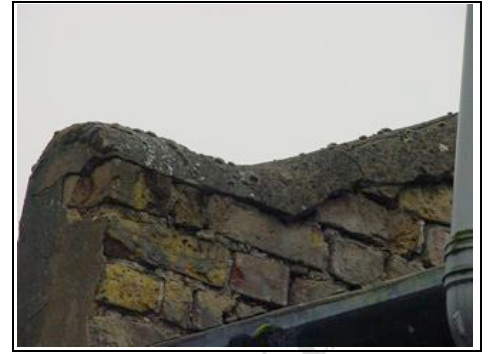
Render coming away and brickwork spalling re-rendering needed
