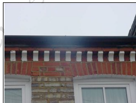
Dog tooth detailing at fascias and soffits
