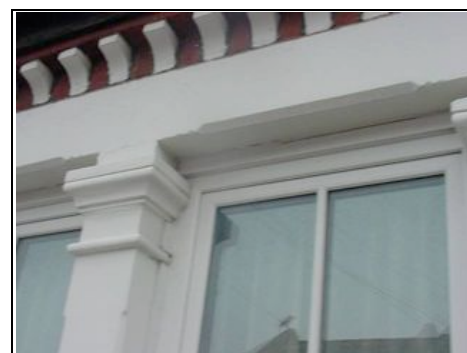
Window without trickle vent
