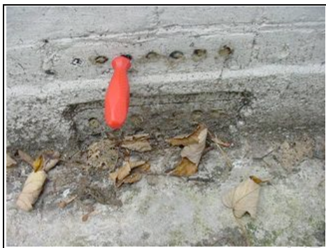
Rear airbricks acting as gutter and also blocked
