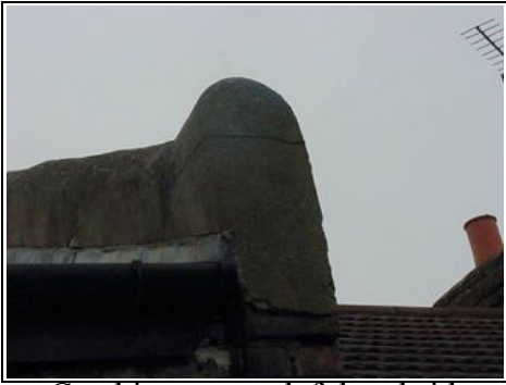
Cracking to rear left hand side parapet wall
