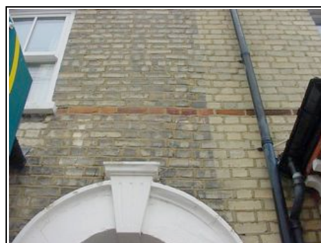
Movement visible to front wall
