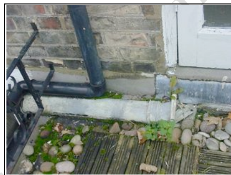
Moss sitting on terrace/balcony due to rainwater sitting on this area.
