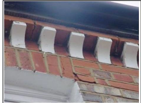
Spalling to soft red brickwork.
