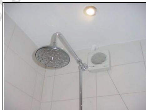
Small extract fan in bathroom
