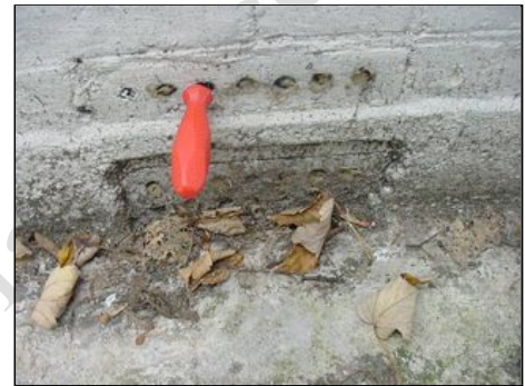
Air brick acting as gutter
