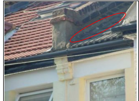
Neighbours side of parapet wall has tile on edge flashing
