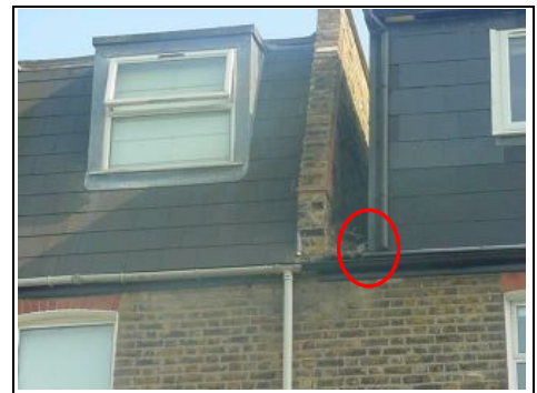
Likely to overflow where down pipe meets gutter
