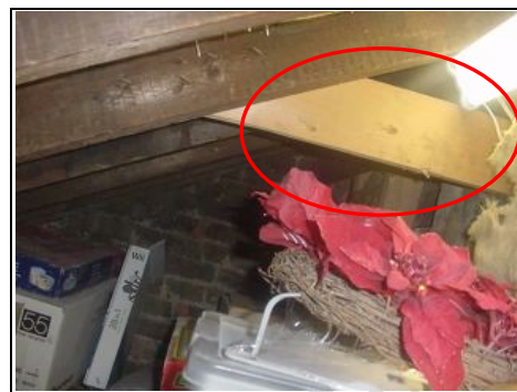
General view of inside of roof with new timbers added
