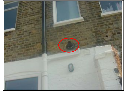
Boiler flue on outside wall
