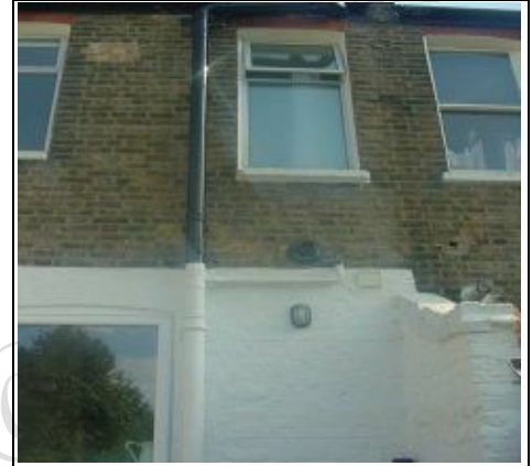
Plastic soil and vent pipe
