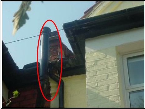
Cast iron soil and vent pipe
