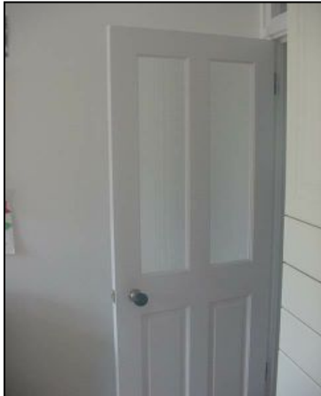
Glazed door to kitchen without safety glass
