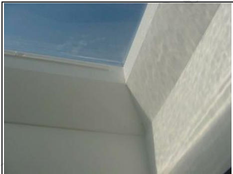
Roof window to flat roof
