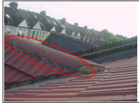
Roof ridge tile is poorly bedded
