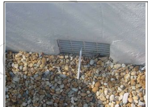
Air brick (front) allow ventilation under floor
