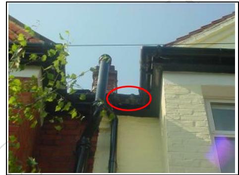
Leaking gutter
