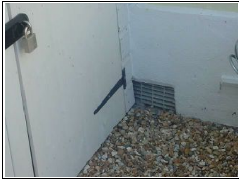
Air brick could be acting as a gutter allowing water in
