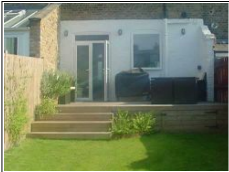
Decking to the rear, we believe, is covering the air bricks
