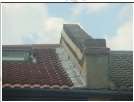
Poor tilting fillet detail to edge of the roof
