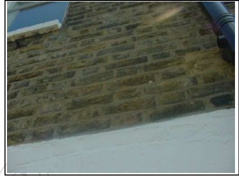
Flemish Bond brickwork
