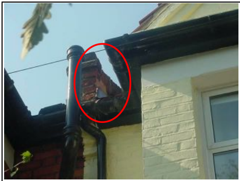
Left parapet wall has not been repaired
