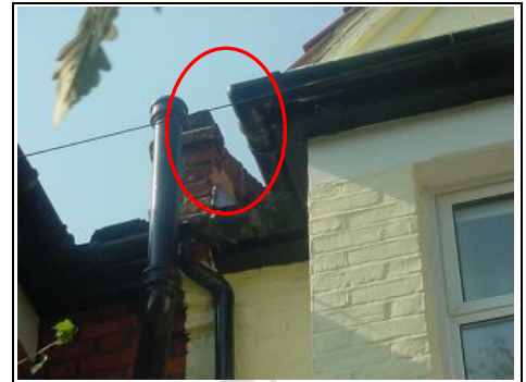
Left parapet wall. We believe this is allowing dampness into the property
