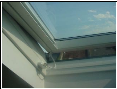
Safety lock on front roof window
