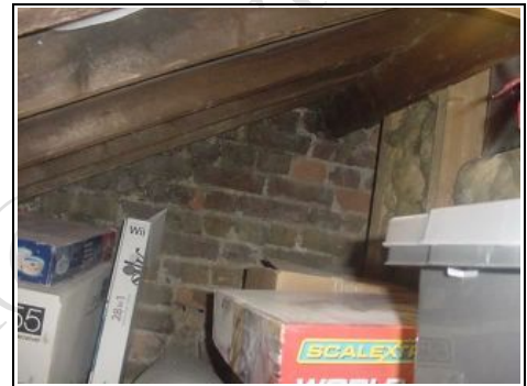
The left hand wall appears to be causing dampness
