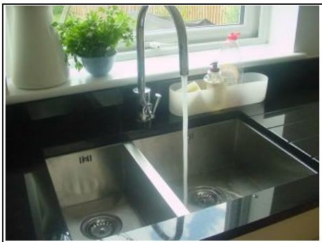
Running the tap checking for back up as no man hole found
