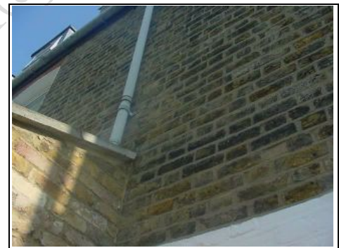
Bricks re-pointed in cement mortar
