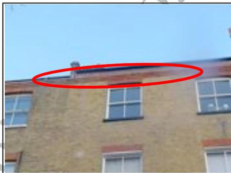
Appears to be deterioration to the red brickwork indicating that the gutter above may be leaking onto it.
