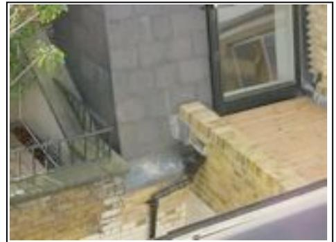
Green moss staining around hopper head indicating it is overflowing
