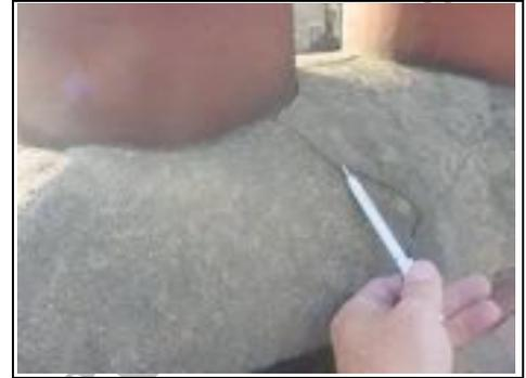
Crack to cement haunching
