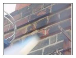
Close up of spalling brickwork
