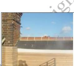
Poor detailing where water will run down the timber and cause pattern staining we believe
