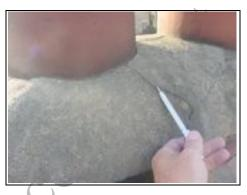
Crack to cement haunching
