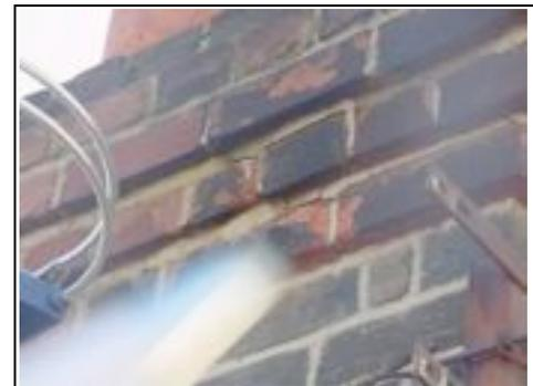
Close up of spalling brickwork
