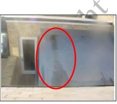
Ponding on single ply roof
