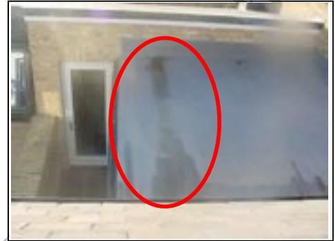
Ponding on single ply roof
