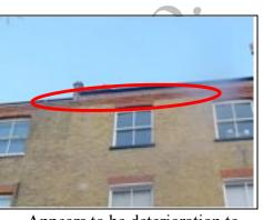
Appears to be deterioration to the red brickwork indicating that the gutter above may be leaking onto it.
