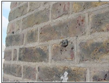
Close up of mortar
