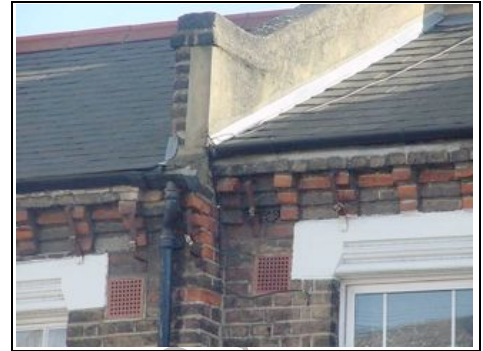
Front left hand parapet wall
