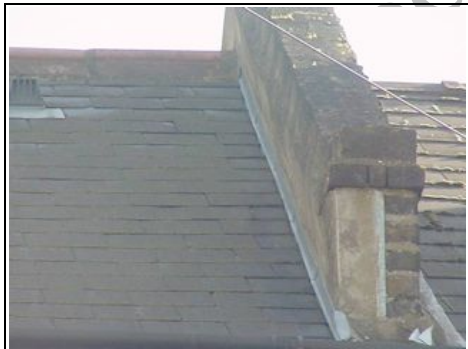
Right hand parapet wall
