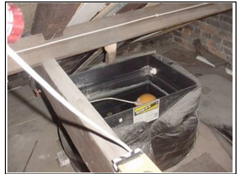
Water tank without lid
