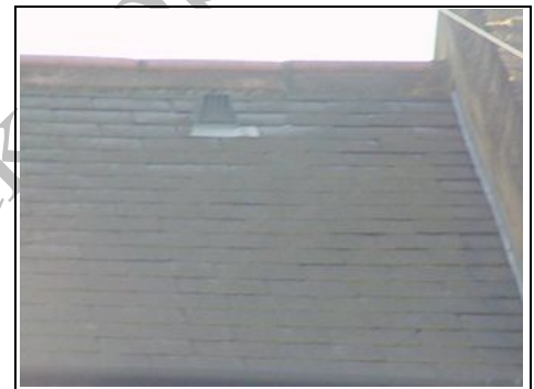
Man made slate roof with vent
