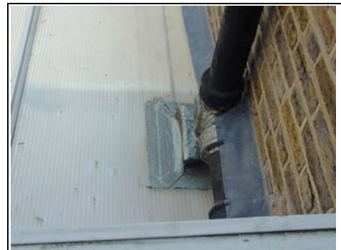
Flashband where it goes into polycarbonate
