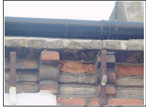
Are these slate guard brackets or electric cable brackets.
