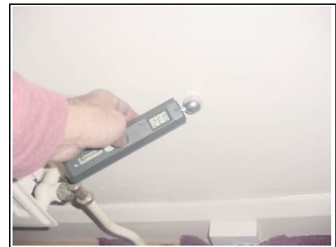
Testing for rising damp
