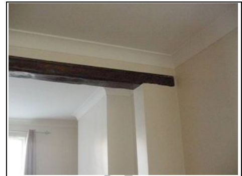
Timber beam to removed wall
