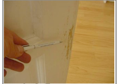
Looks like kitchen door has been attacked by a dog at some point
