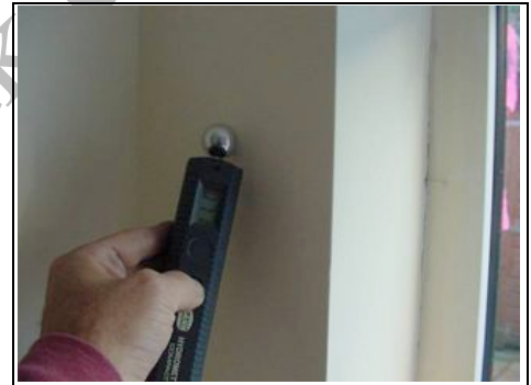
Testing for lateral dampness
