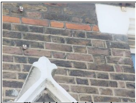
Flemish bond brickwork
