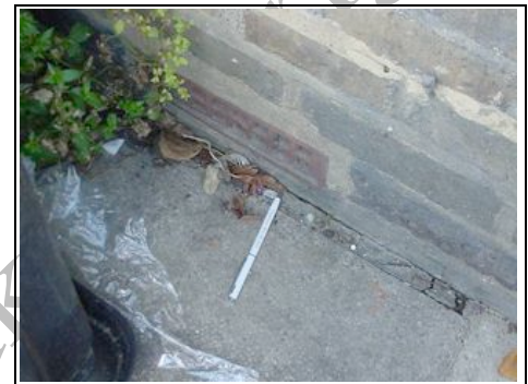
Air brick to front
