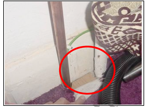
Laminate under carpet under stairs
