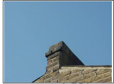
Rear parapet wall
