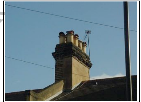
Chimney front left
