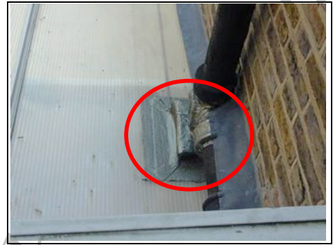
Flashband where it goes into polycarbonate
