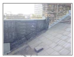
Felt covered parapet wall
