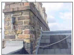
Patch repair and new flashing
