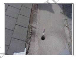
Small opening in valley gutter downpipe
