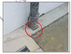
Rodding eye blocked off at base of soil and vent pipe
