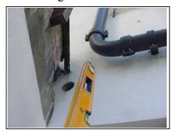
Vertical cracking to rear of the property
