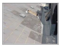
Damaged slate - felt repairs
