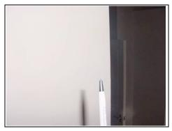
Hairline crack between bathroom and bedroom in top floor apartment – possible sign of movement to the gable end walls.
