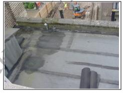
Flat roof - rear Ponding visible
