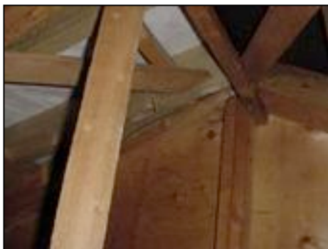
Timber frame construction has been used to form the gable end
