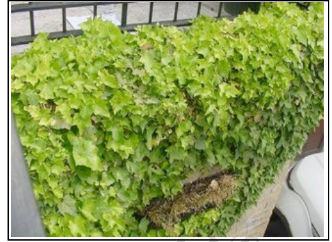
Ivy growing on brickwork
