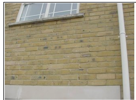
Stretcher bond brickwork
