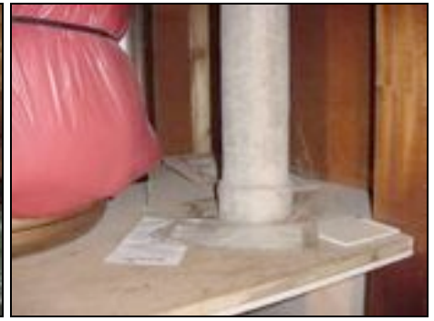
Asbestos found within a 1960's timber frame house
