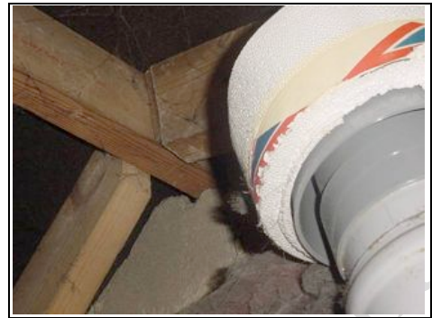
Automatic inlet valve in roof space
