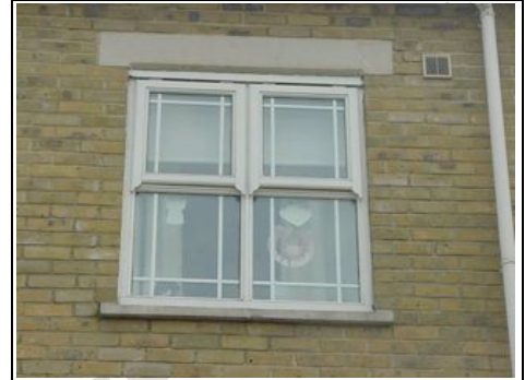
Timber double glazed mock sash windows
