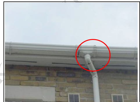
Gutter and downpipe, leaking slightly indicated by staining to the swan neck
