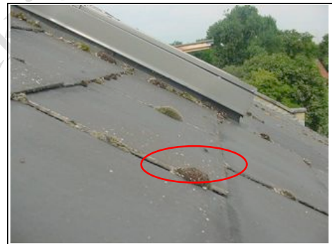
Manmade slate Minor moss visible
