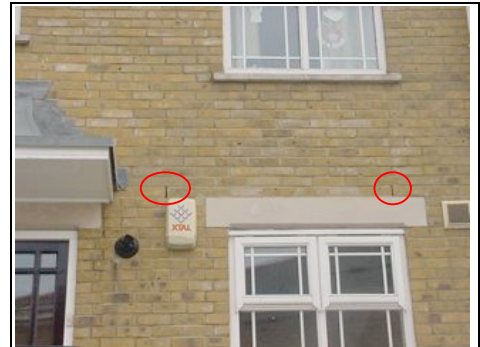
Weep holes above the window
