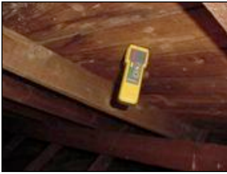
Close boarding to roof of a timber frame house
