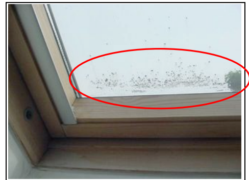
Minor signs of mould
