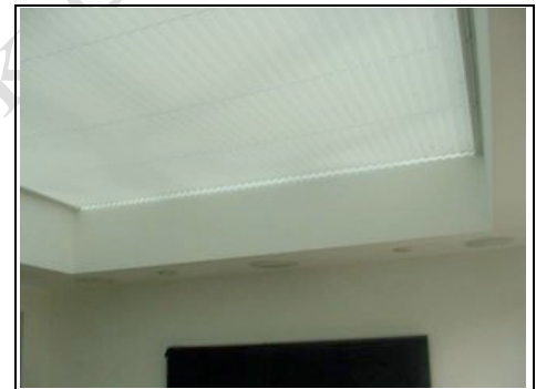
Glazed area of roof can cause heat loss in winter.
