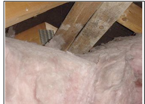
Insulation in the roof space above the shower room
