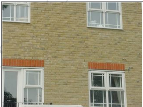
White powdery effect known as efflorescence
