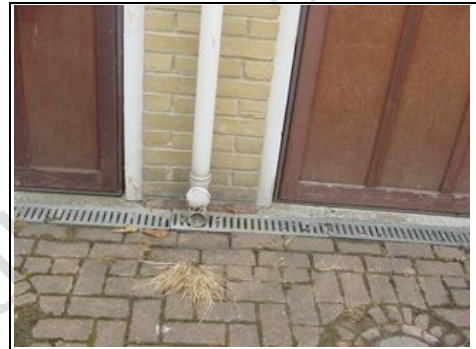
Running gulley to garage
