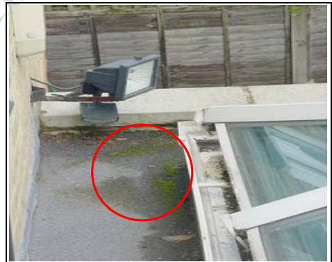
Flat areas on the roof with moss forming
