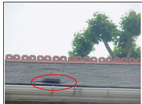
Main roof, manmade slate with tile vent
