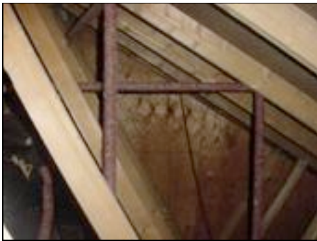
Signs that it is a modern timber framed property – timber found within the roof space
