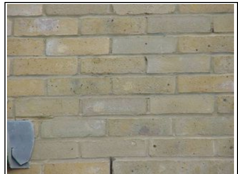
Efflorescence generally to the rear of the property
