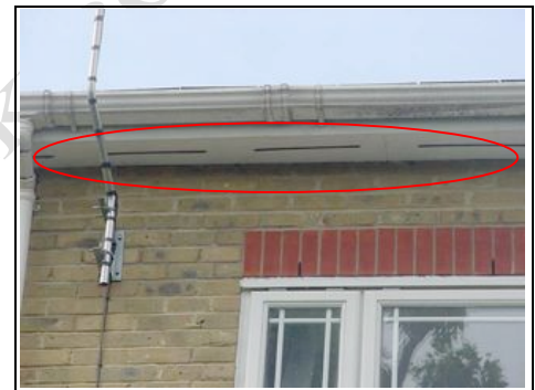
Vented soffit board
