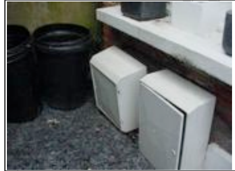
Gas and electric consumer unit to the front of the property
