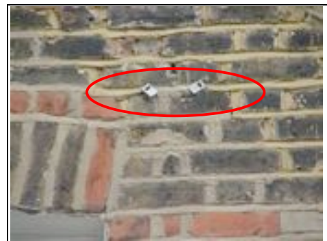
Surveyors 'tell-tale' device for monitoring movement in gable wall
