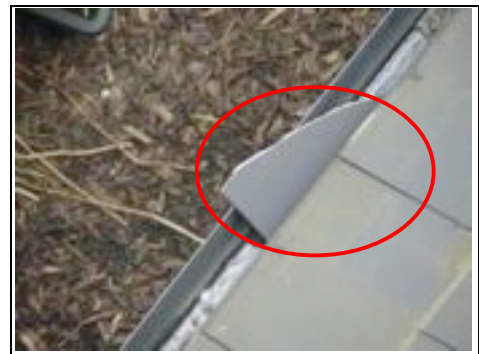
Slipped tile in gutter
