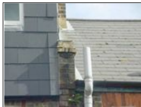
Soil and vent pipe
