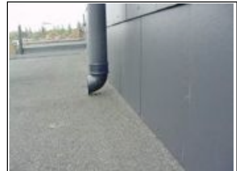
Downpipe discharges rainwater onto the flat roof. A slate should be placed under it.
