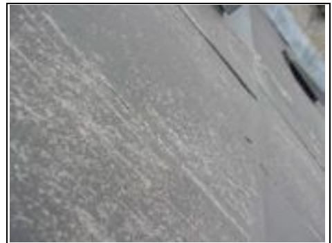
Close up of deterioration on manmade slates
