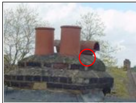
Chimney- rear left Crack in flaunching
