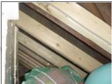
Additional timbers have been added where the room in the roof is
