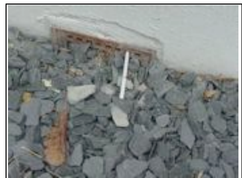
Air bricks to the front are too low and are acting as gutters
