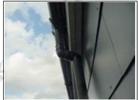
Plastic Gutter and downpipe
