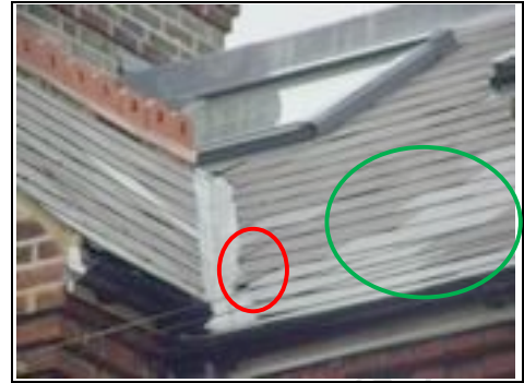
Slipped slates (red) Replacement slates (green)
