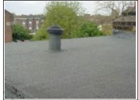
Flue for the soil and vent pipe
