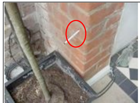
Damp proof course has been inserted vertically as well as horizontally
