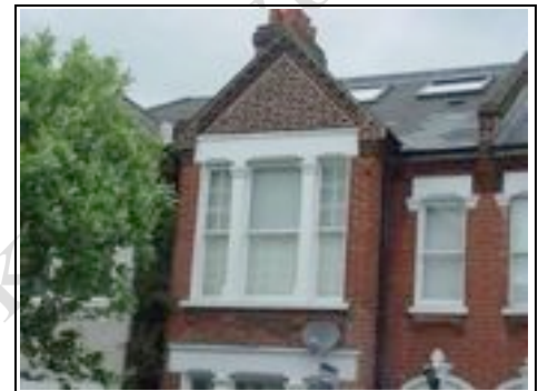
Flemish bond brickwork
