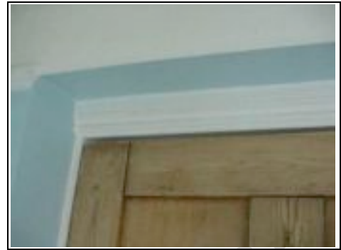
Movement visible in the door of the first floor bathroom
