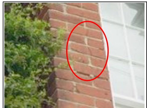
Deteriorating cement mortar visible in wall next to the plant
