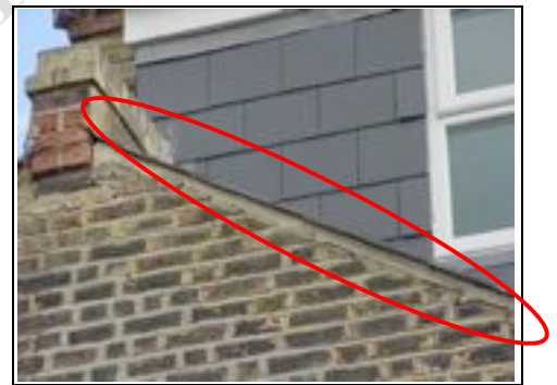
Rear pitched roof to gable wall
