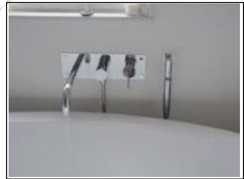
We tend to find this type of shower can leak
