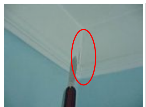
Cracking visible in the bathroom
