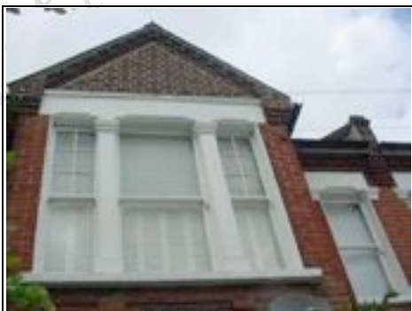
Timber sliding sash window
