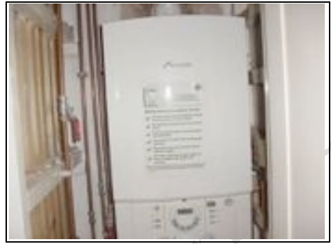
Worcester boiler in bathroom
