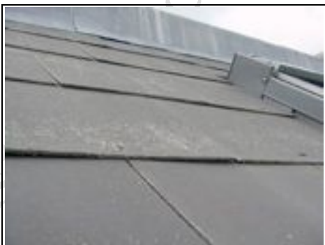
Manmade slates starting to deteriorate
