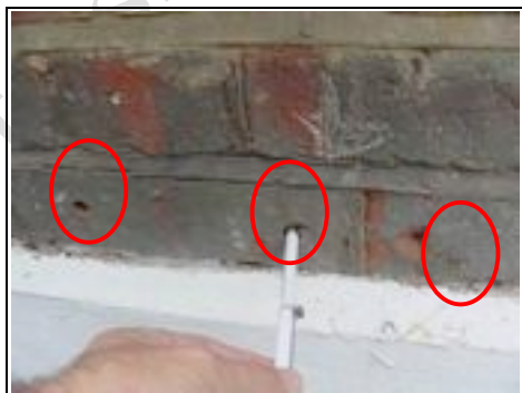
Holes drilled for liquid damp proof course
