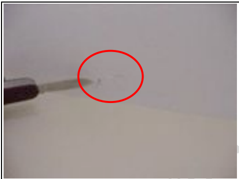
Popping/blistering to the perimeter in second floor bedroom
