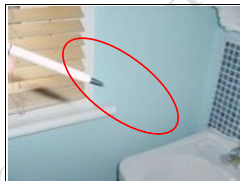
Crack in rear bathroom wall
