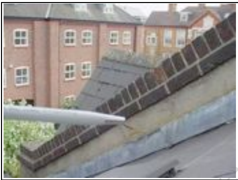
Crack in parapet wall - front left
