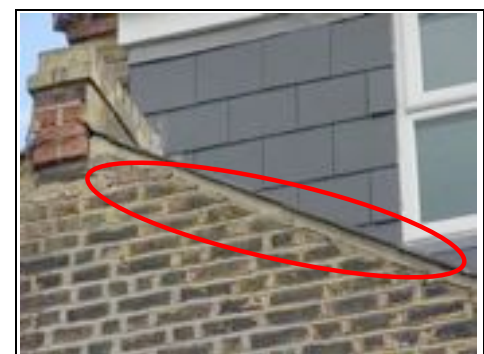
Different colours of cement mortar on rear gable
