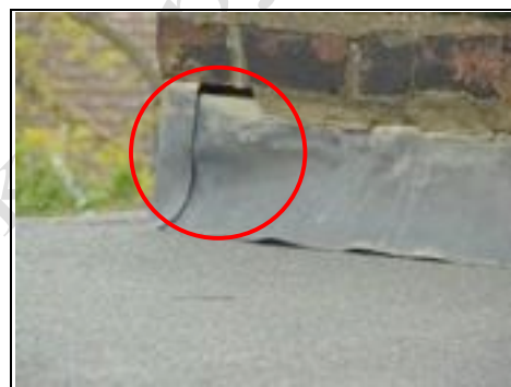
Flashing has not been finished correctly
