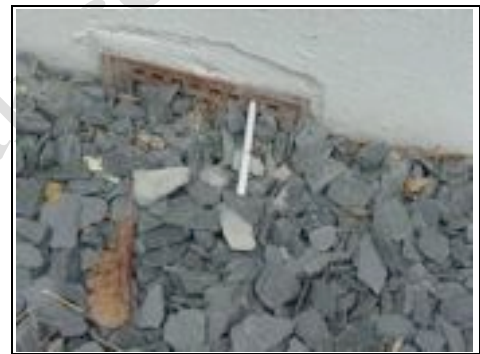
Air bricks to the front are too low acting as gutters
