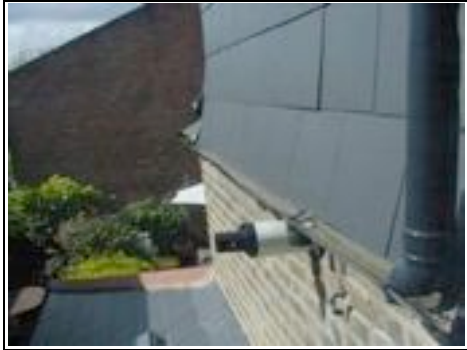
Flue from boiler
