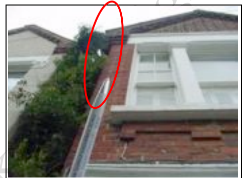
Cracking to front bay area at high level
