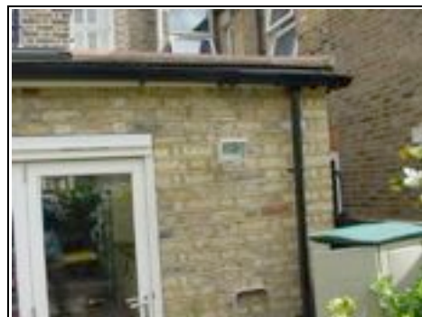
Flemish bond cavity brickwork (assumed)
