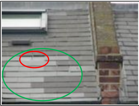
Missing slates (red) Replacement slates (green)
