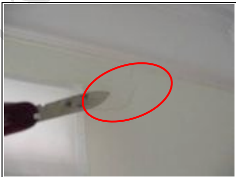
Cracking to the front bedroom on the first floor
