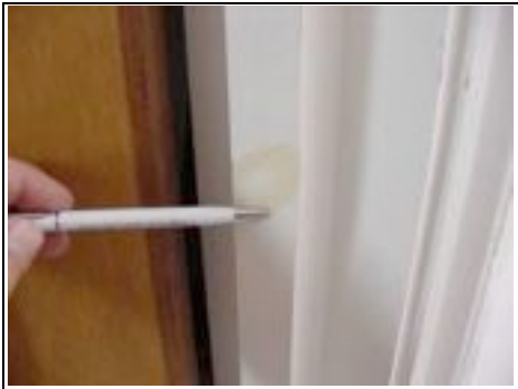
Knots grinning through to door frame in the second floor roof extension
