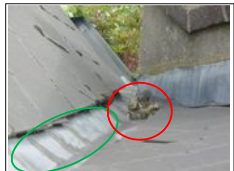
Close up showing cement mortar in the valley gutter (red) Deterioration to valley (green)
