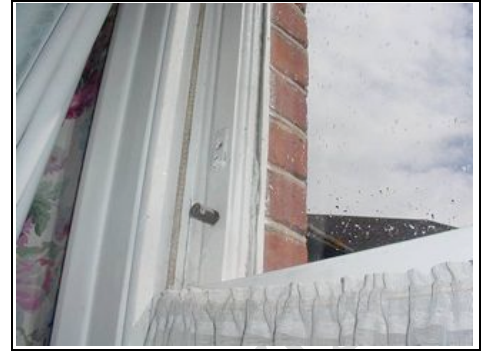
Restrainers on sliding sash window
