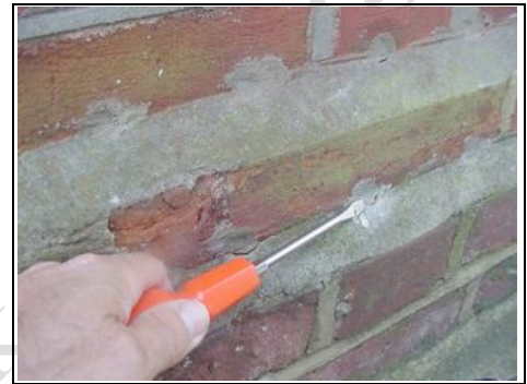
Damp proofing injected twice
