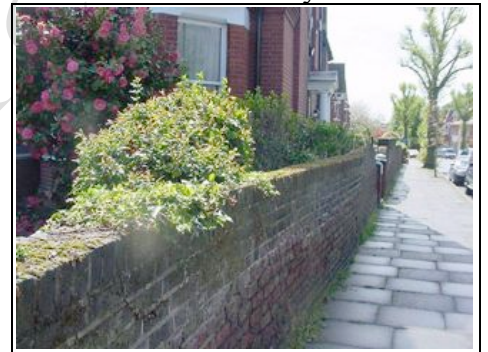
Kink and twist in boundary wall
