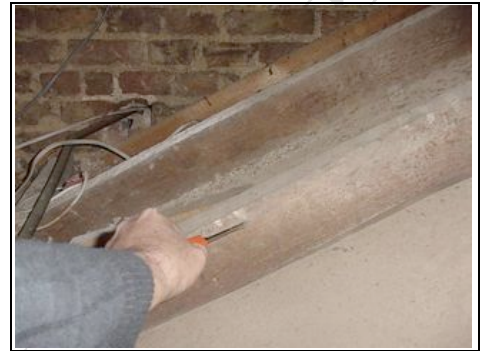
Minor woodworm in roof above the kitchen
