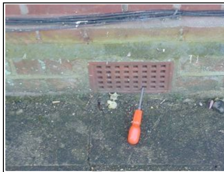
Airbrick acting as a gutter
