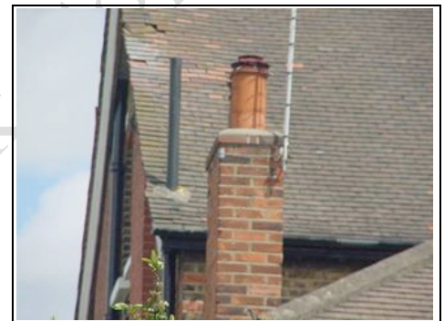
Aerial to chimney
