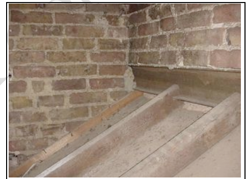
Metal lintel that would have been put in when refurbished
