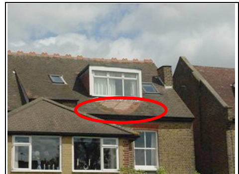
Tiles replaced to base of rear dormer
