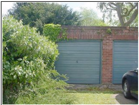
Garage within a block of four
