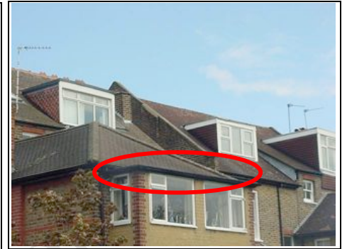
Hipped roof and flat roof (circled to rear bay) to extension
