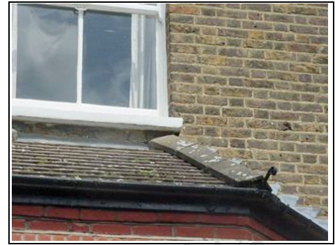
Rear bay window roof
