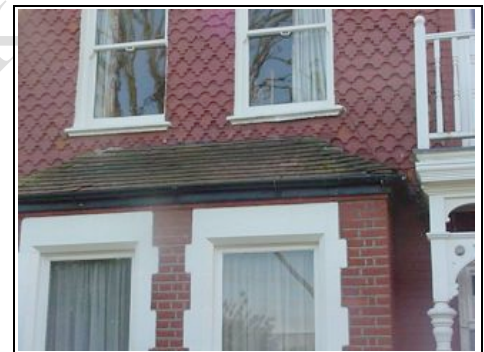
Front left bay roof
