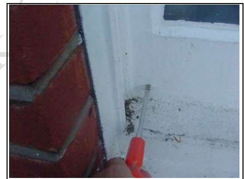
Knife test carried out with screwdriver!
