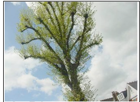
Tree contributing to pushing wall
