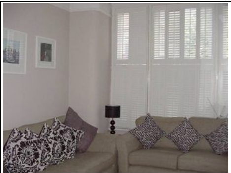
Example of shutters with vents at top open and bottom closed
