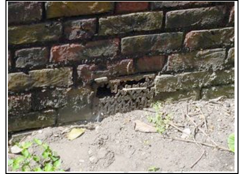
Vent in garden wall
