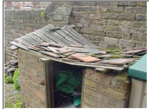
Old coal bunker
