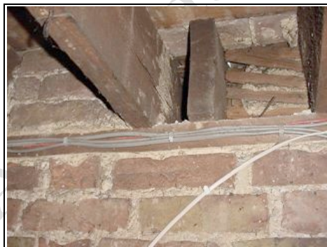
Embedded timbers to first floor above
