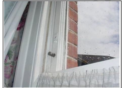
Restrainers on sliding sash
