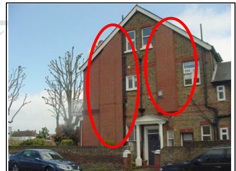
Where chimneys used to be
