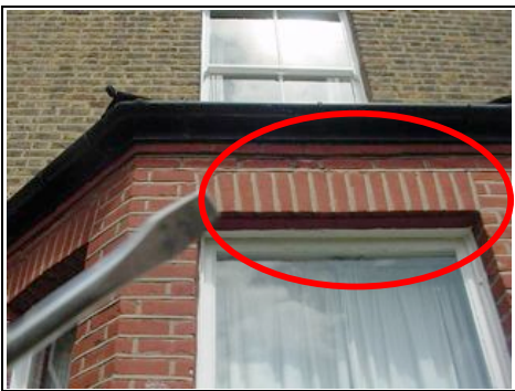
Metal lintel being used under central window of bay
