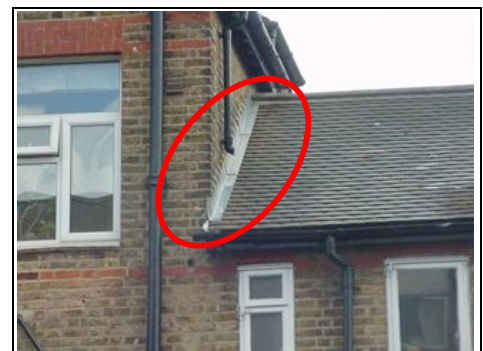
Lead flashing between main building and rear extension 40
