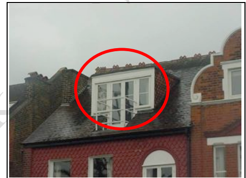
Dormer window to front
