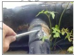
Metal gutter and downpipe to rear deteriorating
