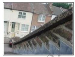
Parapet wall has mortar missing
