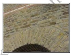
Wrongly repointed in cement mortar
