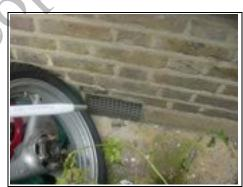
Airbrick acting as gutter
