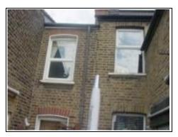
Flemish bond brickwork stitched together indicates some rebuilding has taken place
