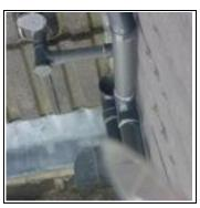
Main roof discharges onto rear roof in one area. There should be wider piece of lead flashing known as deflector
