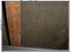
This photo shows the common rafters (the ones that form the pitch of the roof) and the dark area between is the protective underlayer.
