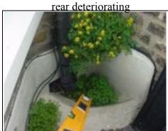
Gulley to downpipes needs clearing
