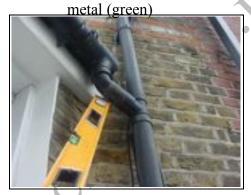
Leaking downpipe to front
