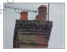
Chimney pot deteriorating which can lead to dampness getting into the property
