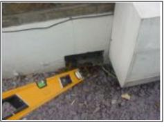
Air brick acting as gutter
