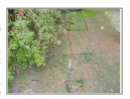
Cracking in rear garden path likely to be from drains
