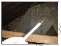
Chimney breast in roof space. Rear chimney has crack in it front, no support can be seen
