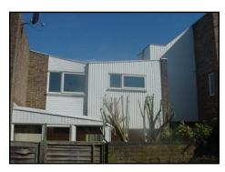
1970's property with cold bridging to the roof beams and the lintels
