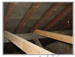
This photo shows the common rafters (the ones that form the pitch of the roof) and the dark area between is the protective underlayer
