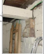
Bricks propping up joist that is holding the floor.
