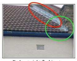
Red – straight flashing to parapet wall Green – stepped flashing to chimney which is how it should be done
