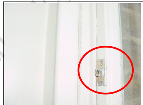
Security locks to windows
