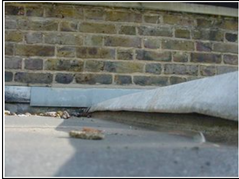
Flat roof above rear right bedroom
