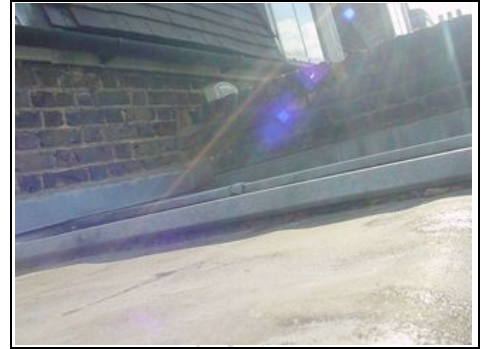
Flat roof above rear right bedroom
