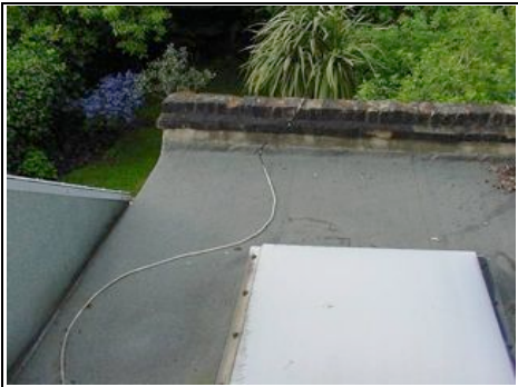
Rear flat roof
