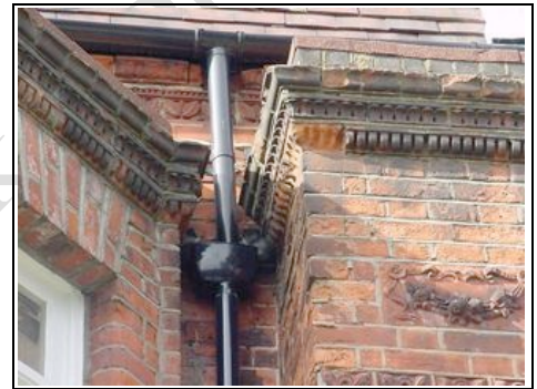
Gutters, downpipes and hopperhead
