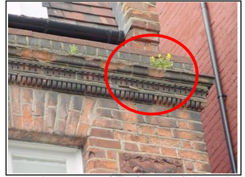
Plants growing from brickwork which is never a good thing
