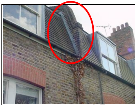
Left parapet wall
