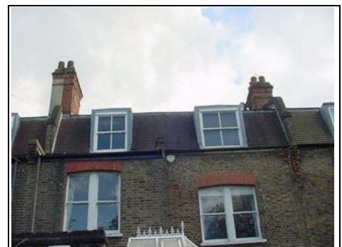
Dormer windows to rear
