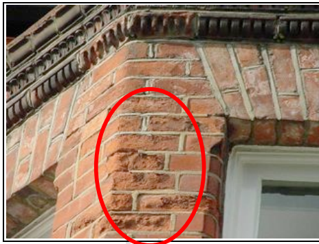
Spalling brickwork
