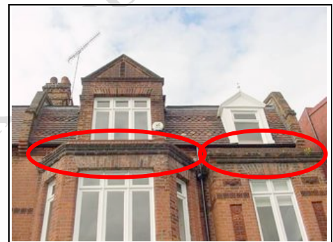
Flat roofs to front bay windows
