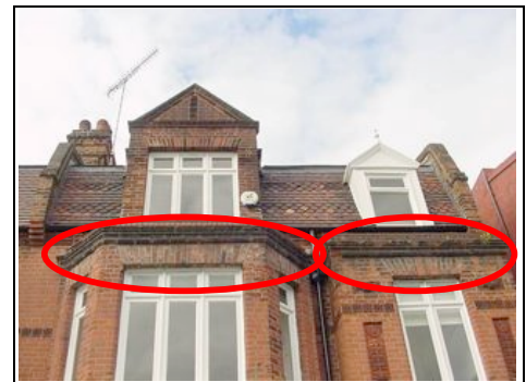
Flat roofs to front bay windows
