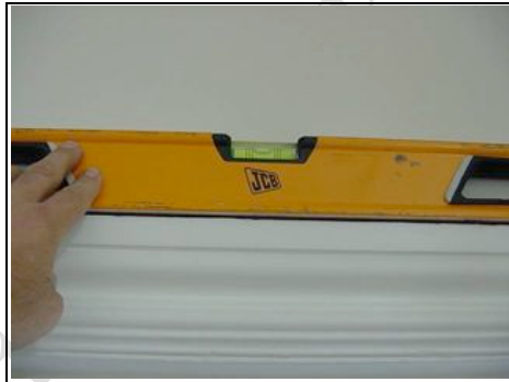
Checking doors are level
