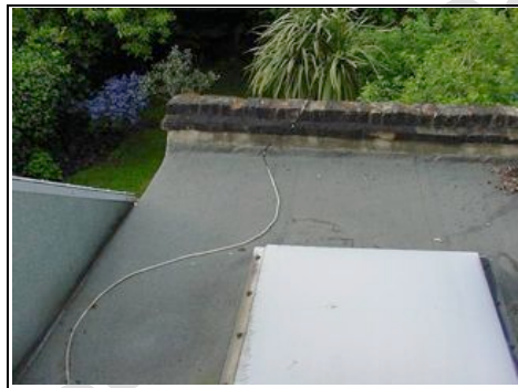
Rear flat roof
