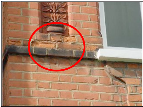
Spalling brickwork
