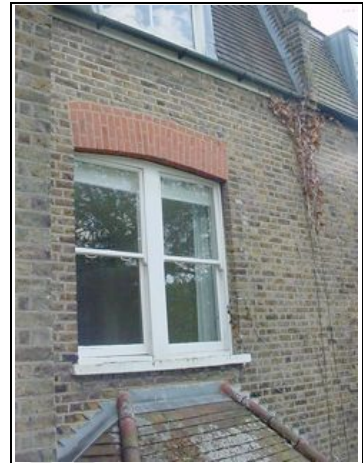
Timber sliding sash windows
