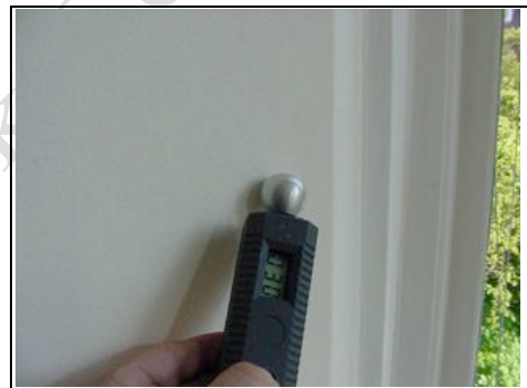
Testing for lateral dampness
