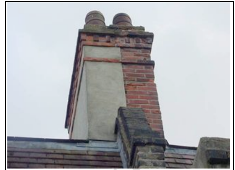
Rear view of Chimney two
