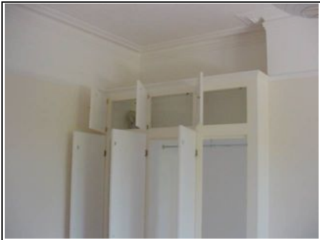
Built in cupboards
