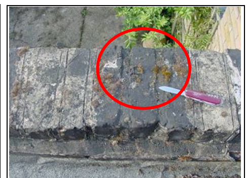
Parapet wall tarred
