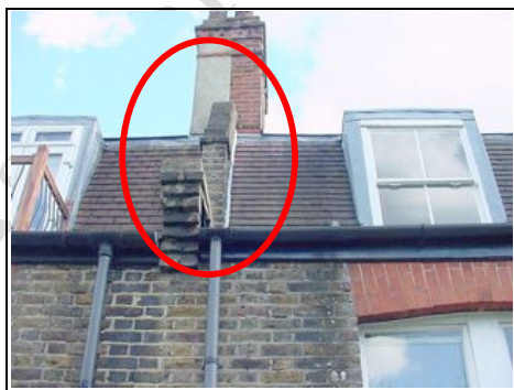
Rear right parapet wall
