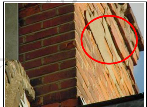
Spalling repaired
