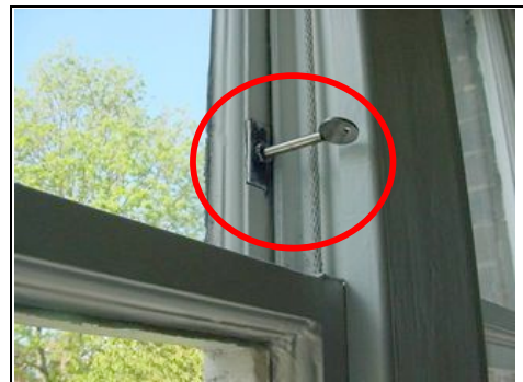
If you turn the key the lock becomes flush
