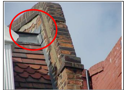
Close up of parapet wall right hand side, rendering to top
