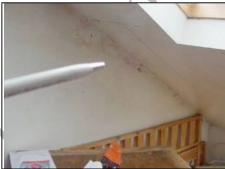
Dampness on front right side from parapet wall
