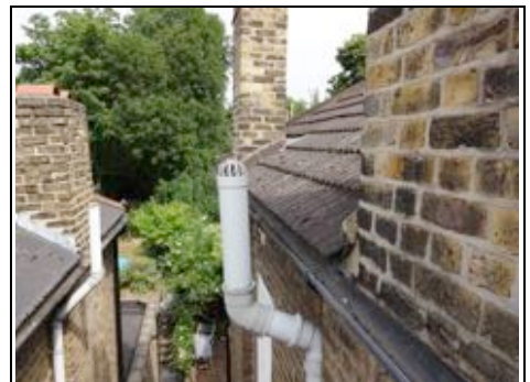
Soil and vent pipe ~ Aerial View - 360 Photo ~
