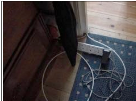
Overloaded electrics – additional socket points required
