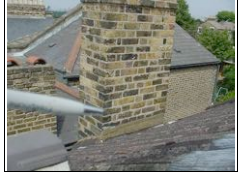
Bottom of chimney –cement flashing?
