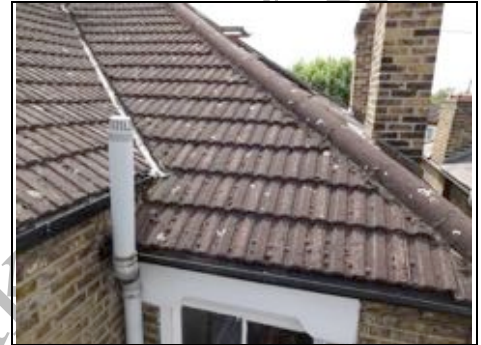
Soil and vent pipe ~ Aerial View - 360 Photo ~
