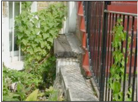
Awkward detail that we believe is allowing dampness into ground floor flat
