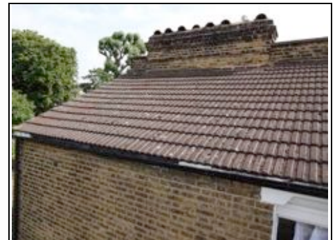
Rear chimney – replace flashing with lead flashing ~ Aerial View - 360 Photo ~
