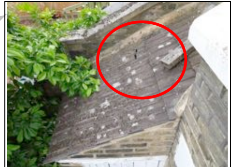
Crack in tile ~ Aerial View - 360 Photo ~
