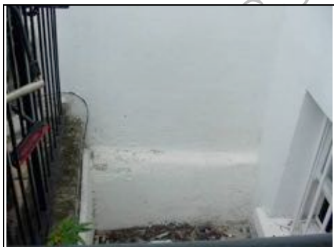
Flaking paint indicating dampness in lower ground floor flat
