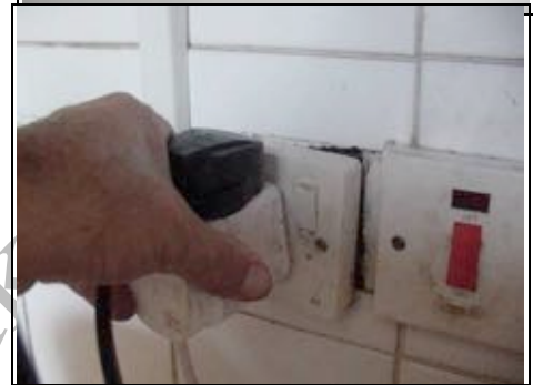
Some socket points not secured
