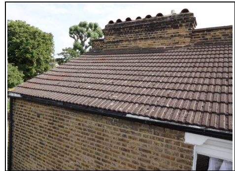
Rear right chimney closed with the hog back tiles
