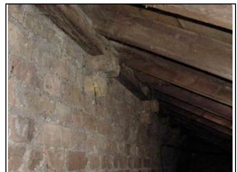
Timber wall plate in rear right roof
