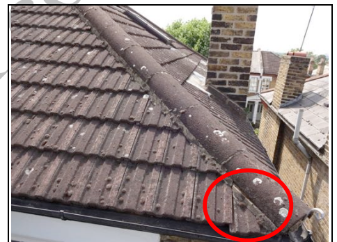
A tile has moved on the corner of the property
