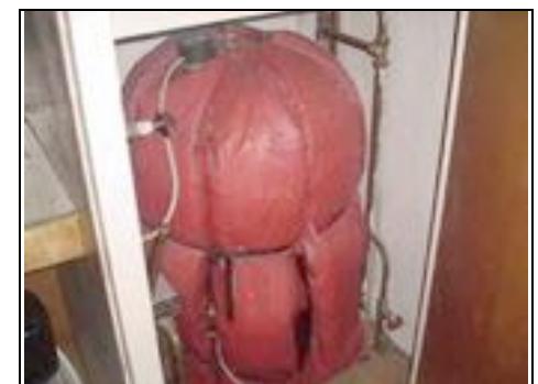
Older style cylinder with loose insulation jacket
