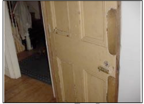
Damage and wear to doors
