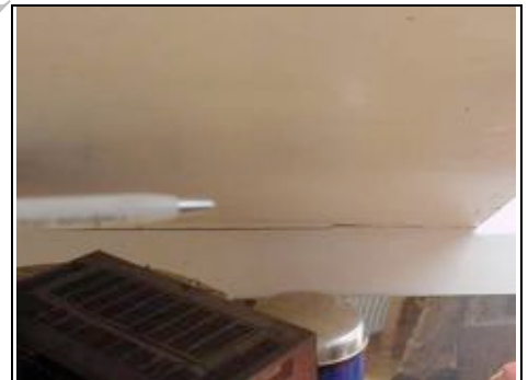
Straight line plasterboard cracking in room in the roof
