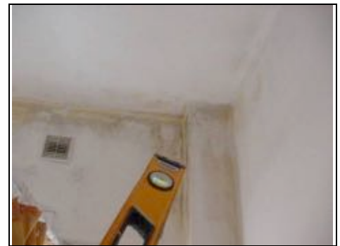
Mould in bathroom
