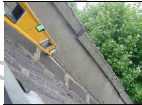
Tile on edge to the Front Right Parapet wall
