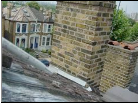
Front chimney has flashband repair to rear
