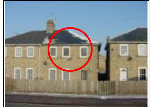
Inappropriate double glazed windows change the look of the property Red circle is insulated roof indicated as snow is not visible
