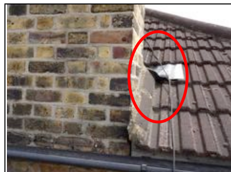
Tile on end to chimney ~ Aerial View - 360 Photo ~
