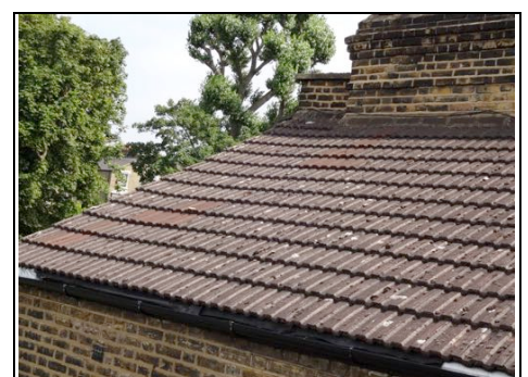
Some tile replacement to rear of roof ~ Aerial View - 360 Photo ~
