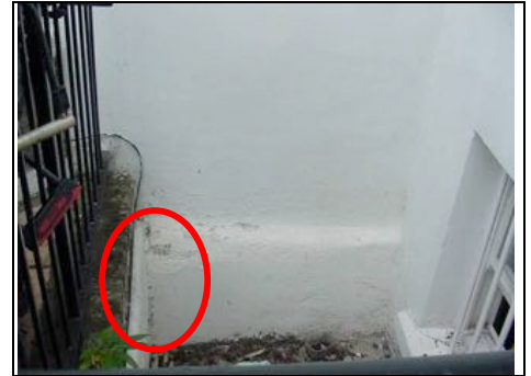
Dampness in lower ground floor
