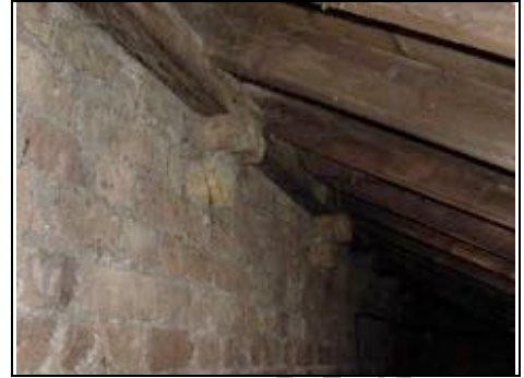
Wall plate deteriorating
