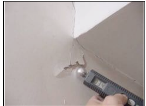
Skin coat of plaster breaking up
