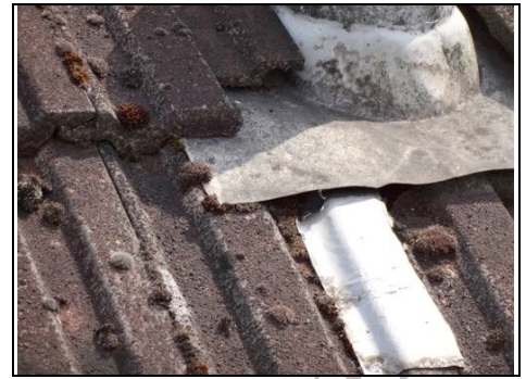
Dampness is getting in around the flue ~ Aerial View - 360 Photo ~
