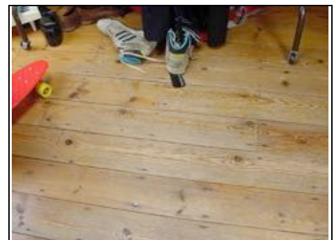
Exposed wood floor show joists are running from side to side
