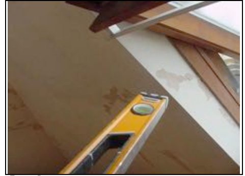
Paint coming off in room in roof
