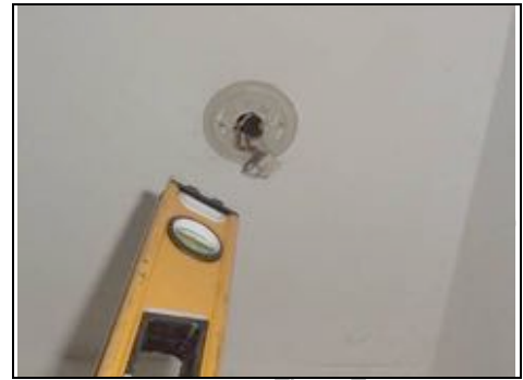
Smoke alarm removed
