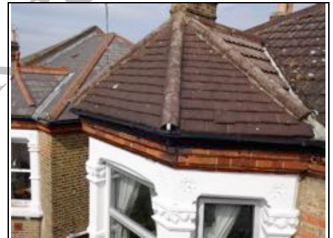
Hipped roof above splayed bay to front has smaller concrete tile ~ Aerial View - 360 Photo ~
