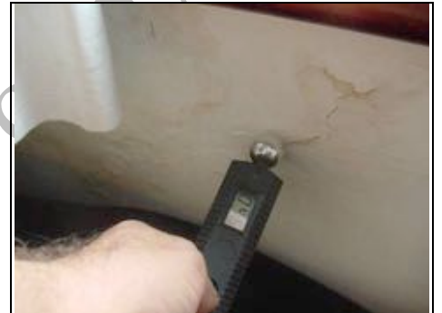
Dampness in front bay window probably wind driven rain or may be condensation
