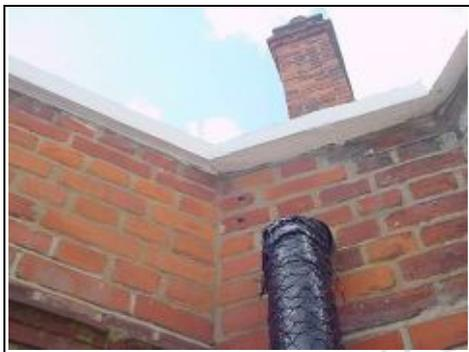
Parapet wall with box gutter behind it. The different brickwork indicates it has been rebuilt
