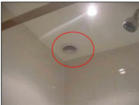
Small extract fan in en suite should be replaced with large humidity controlled extract fan
