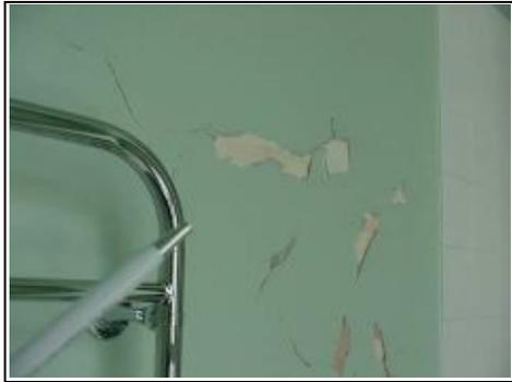
Condensation causing the paint to peel
