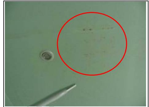
Mould and staining to the ceiling
