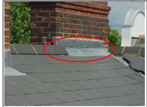
Poor quality flashing around chimney
