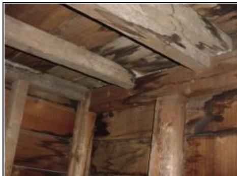
Flat roof to fire escape is allowing water in
