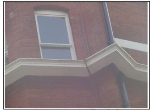
Pointing has weathered to the left hand side of the downpipe
