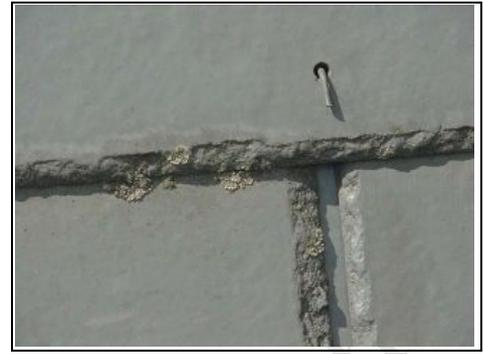
Pins facing down instead of upwards
