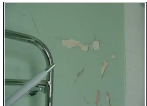
Condensation causing the paint to peel in the bathroom
