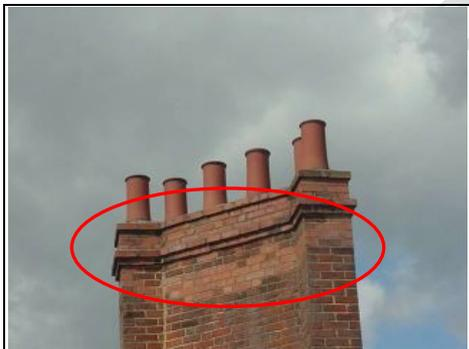
Where we believe the chimney has been rebuilt
