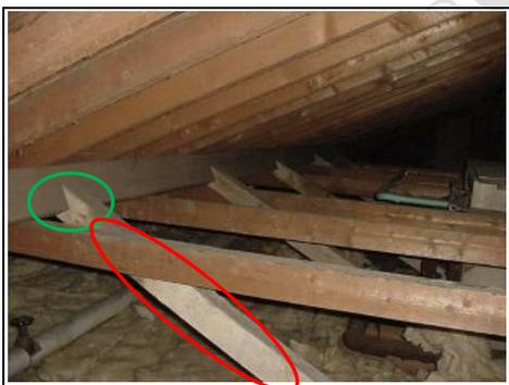
Extra timbers/struts (red) have been added in to the purlins using a bird mouth cut (green)
