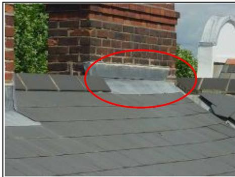
Flashings around chimneys where dampness is getting in. These look to have been replaced but the quality looks poor
