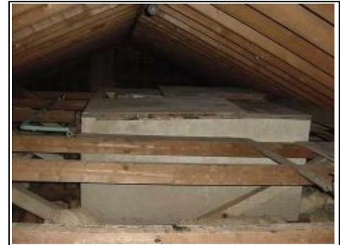
Possible asbestos clad water tank
