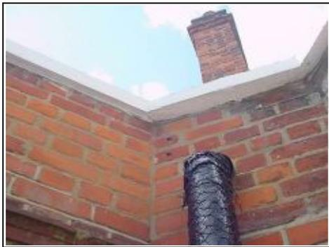
Parapet wall with box gutter behind
