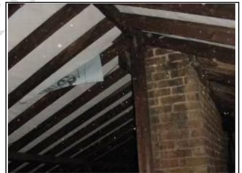
Dampness coming in near the chimney in this roof
