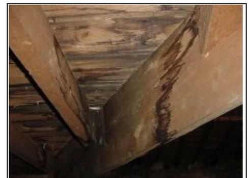
Dampness coming in to the relatively modern flat roof extension for the fire exit
