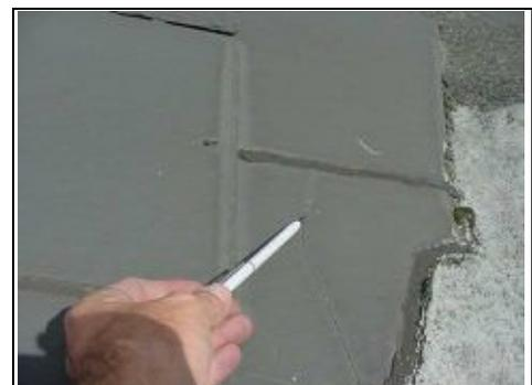
Mastic roof repair between the slates above the kitchen area
