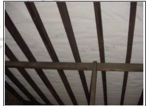
This photo shows the common rafters (the ones that form the pitch of the roof) and the light area between is the protective underlayer.
