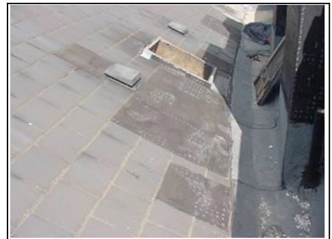
Damaged slate – felt repairs
