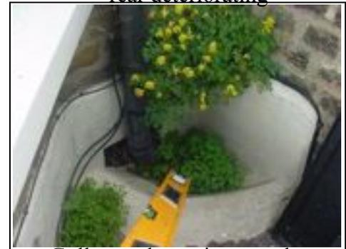
Gulley to downpipes needs clearing
