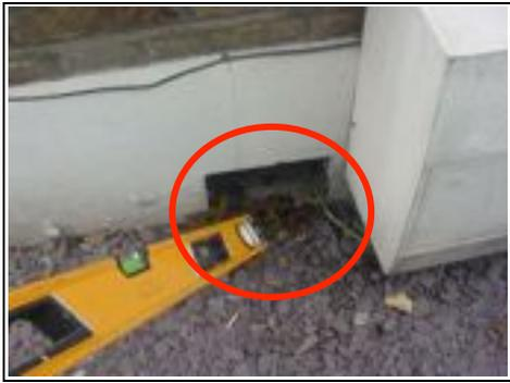
Airbrick acting as gutter
