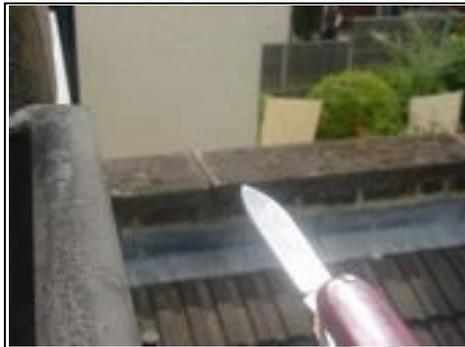
Mortar missing between coping stones
