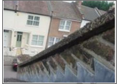
Parapet wall has mortar missing
