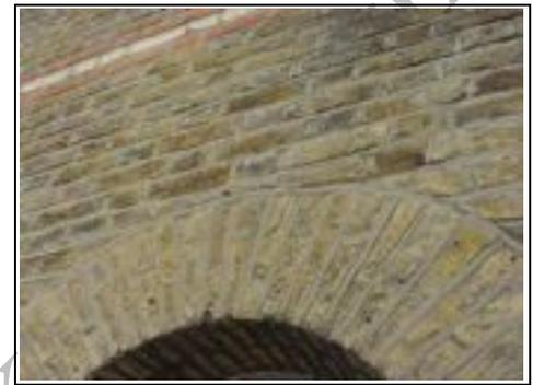
Wrongly repointed in cement mortar
