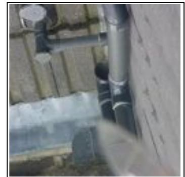
Main roof discharges onto rear roof in one area. There should be wider piece of lead flashing known as deflector
