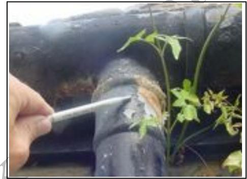
Metal gutter and downpipe to rear deteriorating
