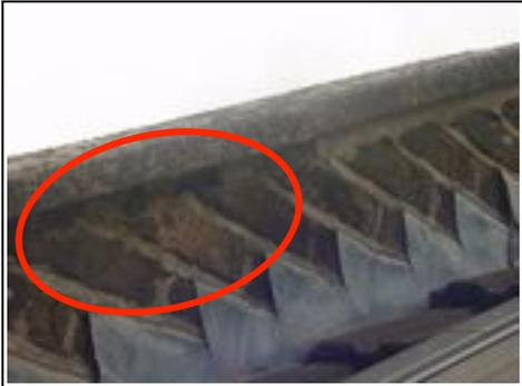
Mortar missing under coping stones
