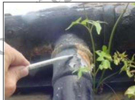
Metal gutter and downpipe to rear deteriorating
