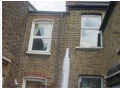
Flemish bond brickwork stitched together indicates some rebuilding has taken place
