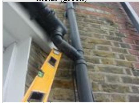
Leaking downpipe to front
