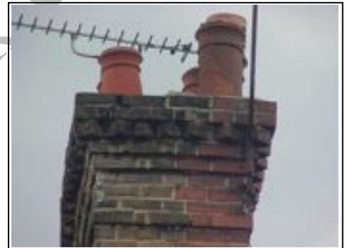
Chimney pot deteriorating which can lead to dampness getting into the property
