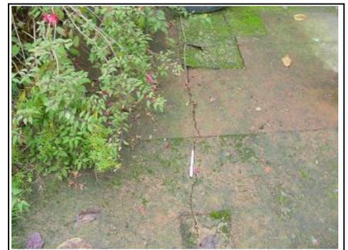
Cracking in rear garden path likely to be from drains
