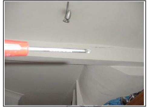
Crack in beam in kitchen
