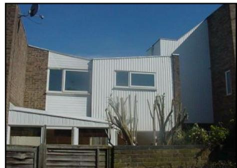
1970's property with cold bridging to the roof beams and the lintels
