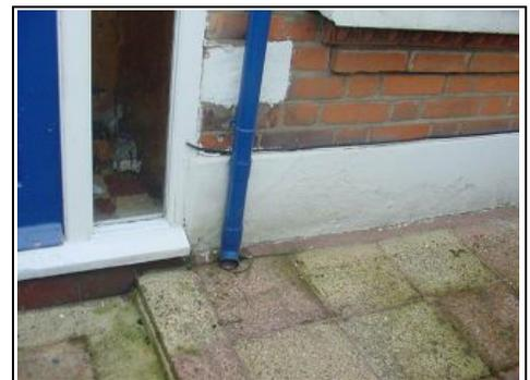
Downpipe discharging onto ground
