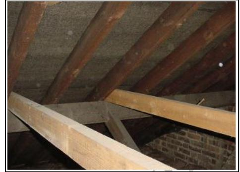
This photo shows the common rafters (the ones that form the pitch of the roof) and the dark area between is the protective underlayer
