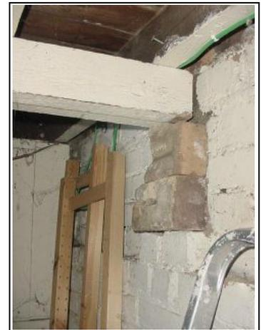
Bricks propping up joist that is holding the floor.
