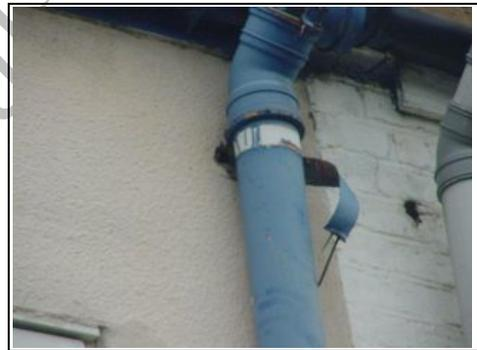
Securing bracket coming away from soil and vent pipe
