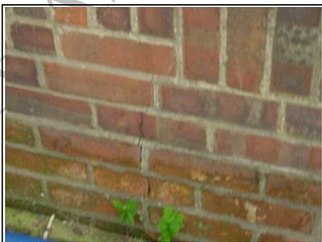
Cracking to front wall
