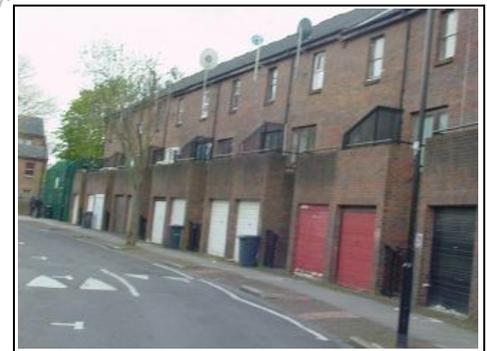
1960's properties built with concrete lintels that can cause Cold Bridging
