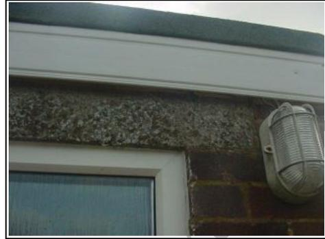
A close up view showing there is a concrete lintel over the door and window.
