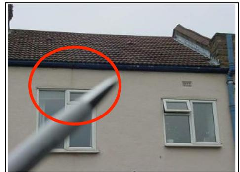
Leaking gutters to rear
