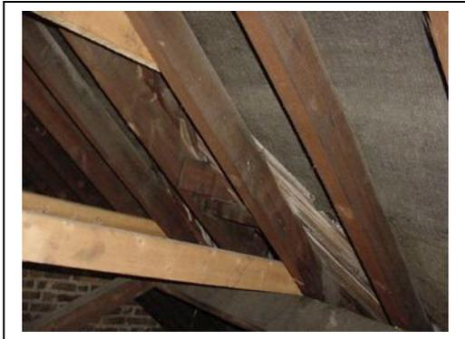
Leaking valley gutter
